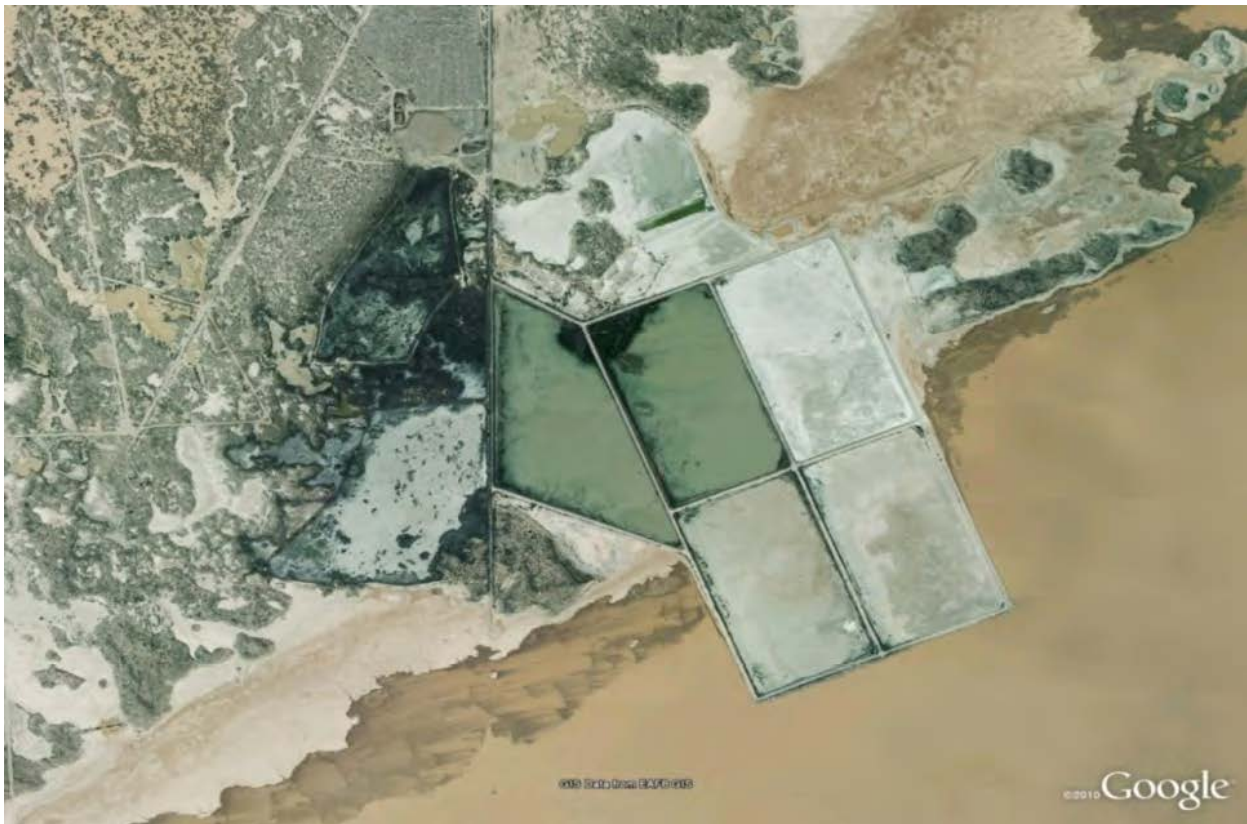
Old and current South Base WWTP evaporation ponds
