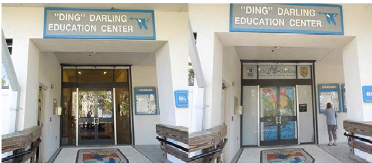
A bird friendly film was applied at the entrance of the Ding Darling Education Center at the J. N. "Ding" Darling National Wildlife Refuge. Photo shows entrance before (left) and after (right) application. Photos by USFWS
