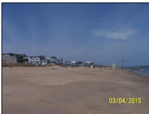
Figure 22. Residential area adjacent to the northern boundary of Virginia Army National Guard – Camp Pendleton
