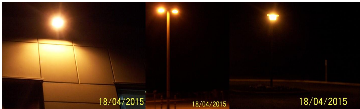
Figure 8. Examples of high-pressure sodium lamp light sources at Naval Air Station Oceana – Dam Neck Annex
