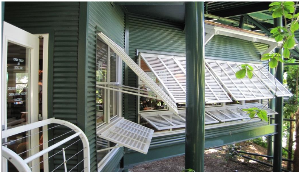
Shutters overhang windows at a facility at the San Diego Zoo. Photo by Christine Sheppard, ABC
