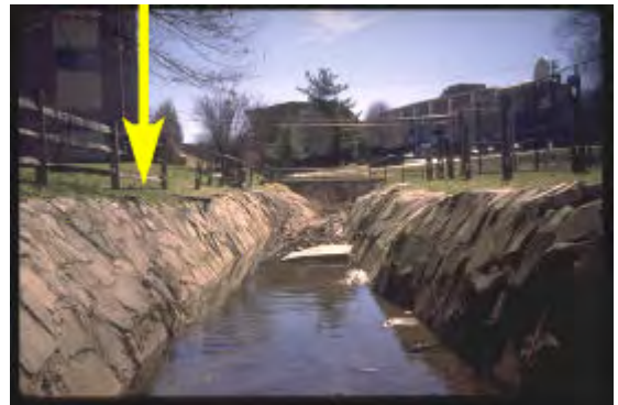
Poor Range (arrow pointing to channelized streambank with no vegetative cover) (MD Save Our Streams)
