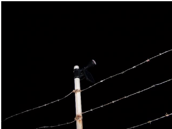
Figure 21. Solar-powered light-emitting diode lamp installed on the northern boundary fence of Virginia Army National Guard – Camp Pendleton
