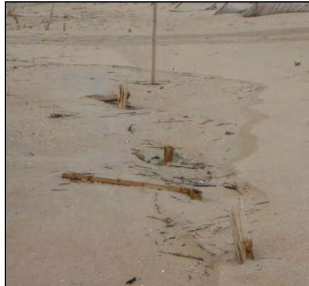
Dune fencing damage post Hurricane Sandy
