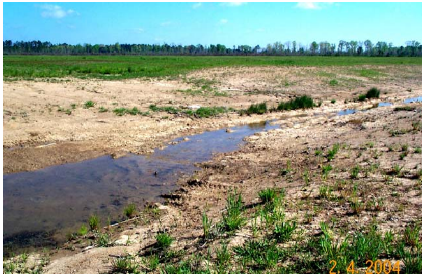
Before picture of Shuqualak Creek erosion
