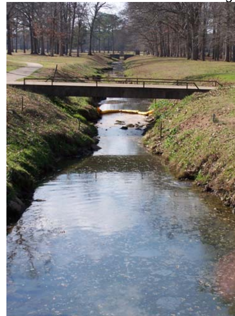
Boom installed on far side of bridge restrains runoff from flightline.
