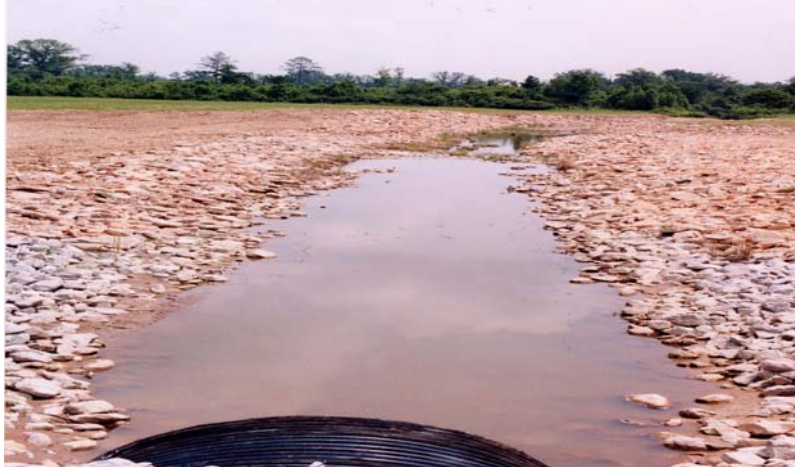
Shuqualak Creek after erosion control installed
