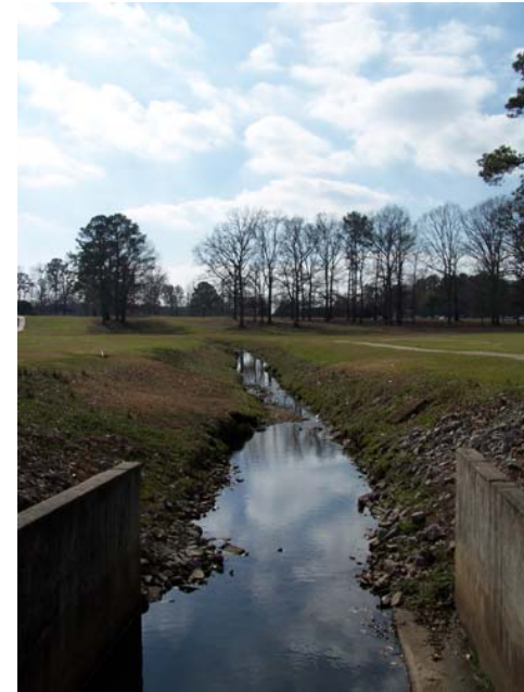
Runoff from the airfield drains through the golf course.
