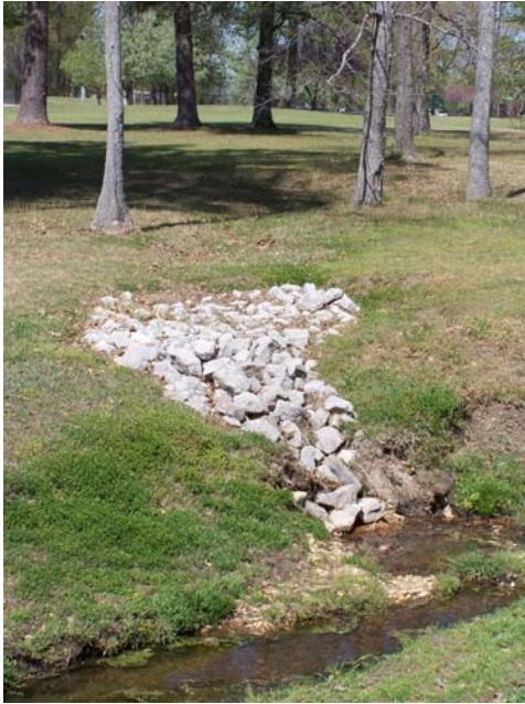
Erosion control measures are implemented as needed.
