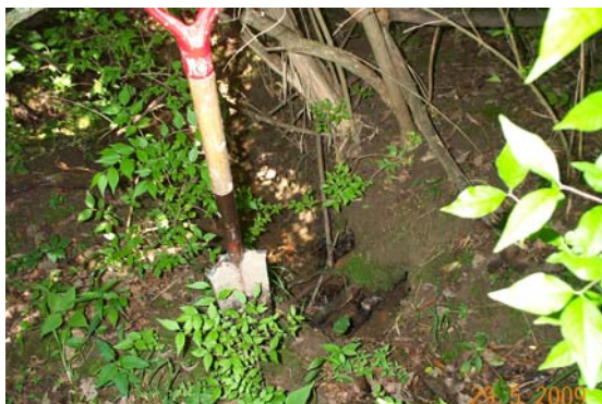
Photo 3 Tile exposed tile outlet from swale
