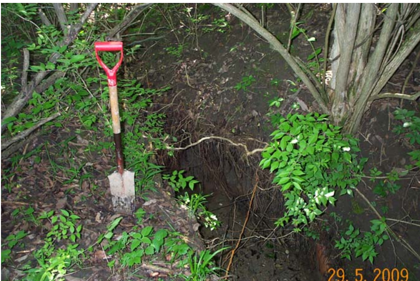
Exposed drainage tile & associated head-cut outlet.
