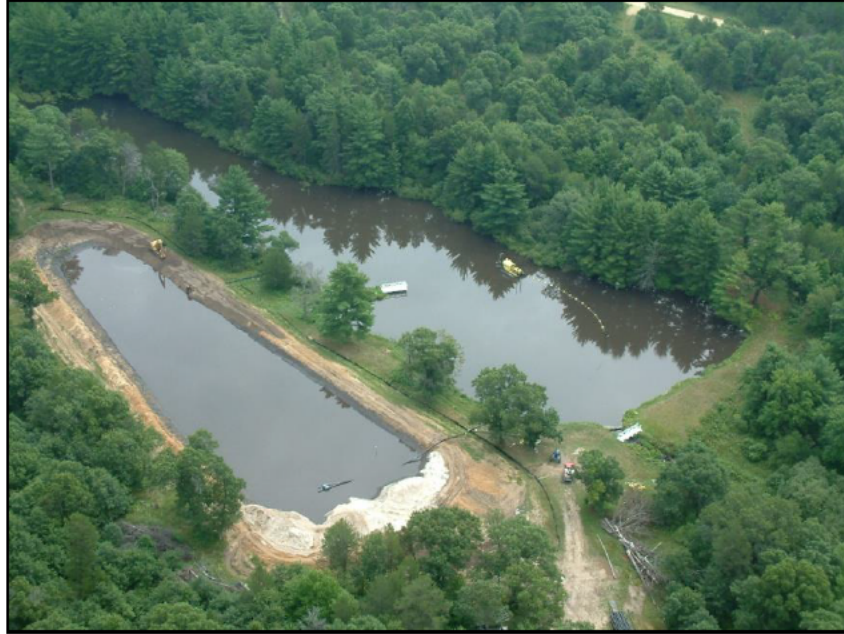
Figure 7. Dredging operations on Hazel Dell Lake.
