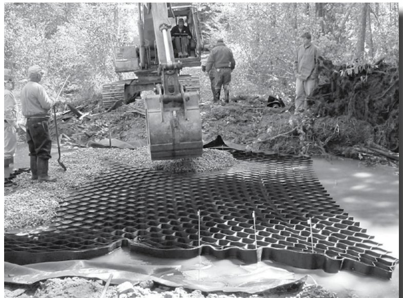
Installation of a Geo-Web® hardened ford.
