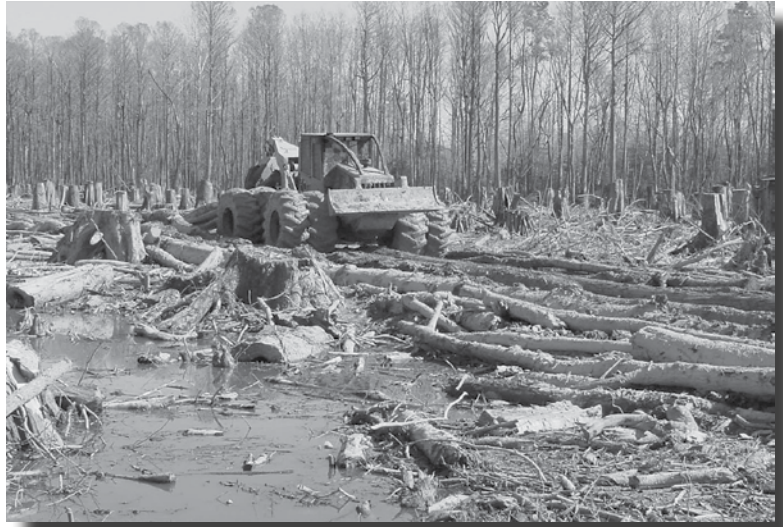
Poor wetland logging practice
