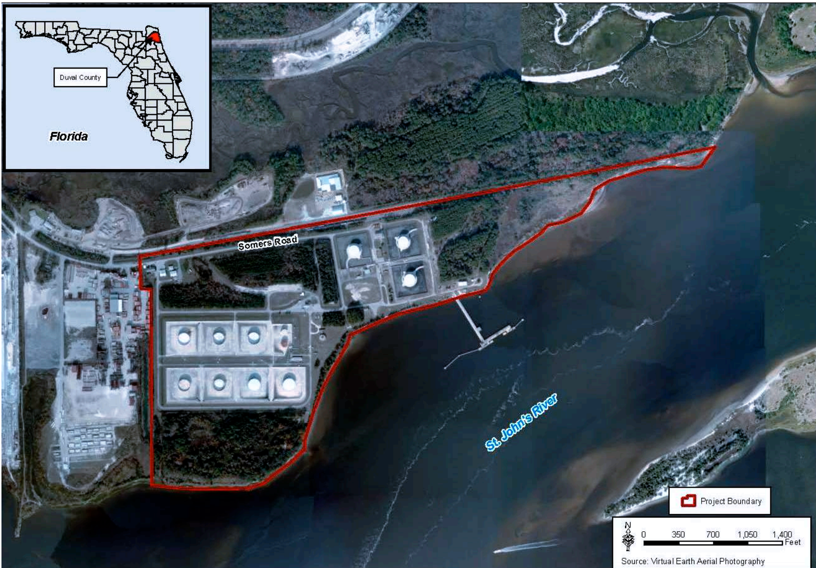
Figure 2-2. Base Map of Fleet and Industrial Supply Center Jacksonville Navy Fuel Depot (NFD).
