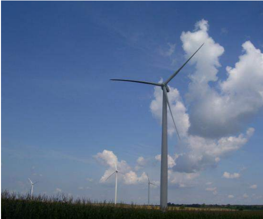
Wind turbines adjacent to the MTC along N 23 rd Road
