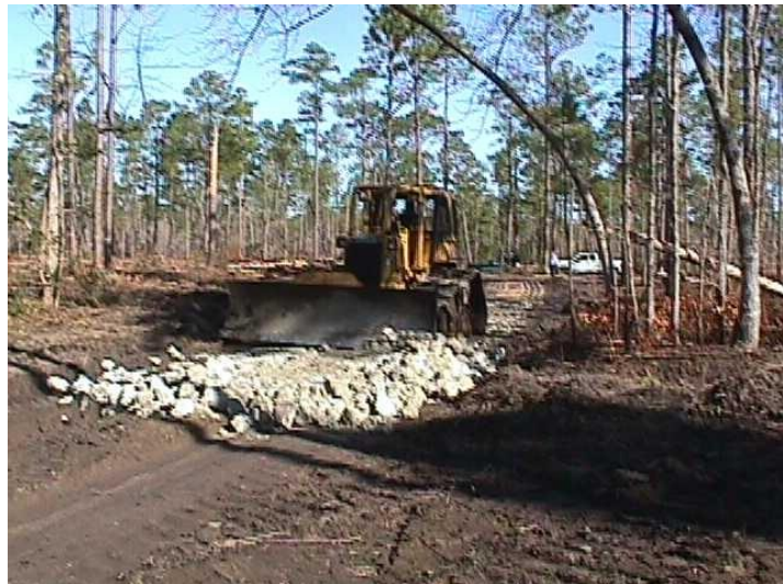
Figure 12. Forest access road repaired by Base Forestry personnel.
