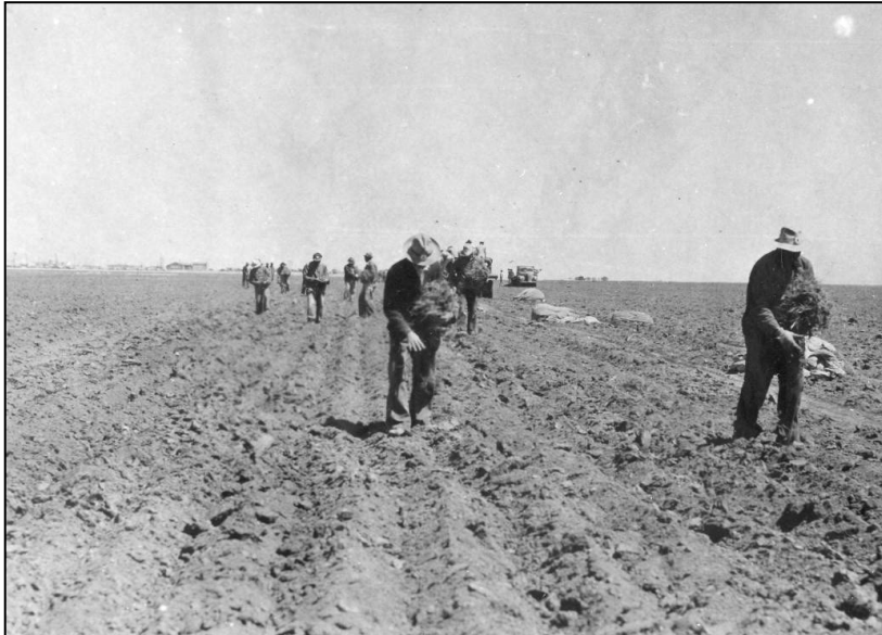
Early Construction of Tinker AFB: Workers sprigging airfield with exotic Bermuda grass in 1941.
