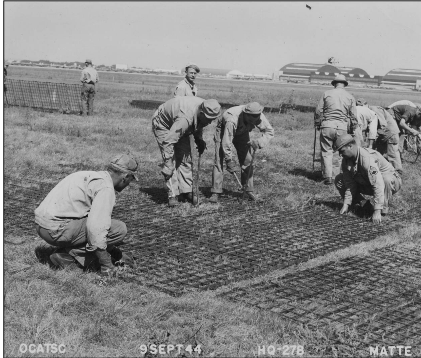
Tinker Airfield: Metal runway matting placed on vegetated areas of the airfield in 1944.
