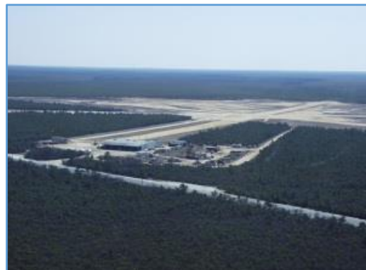
The construction of WGR Photo from WGR archives
