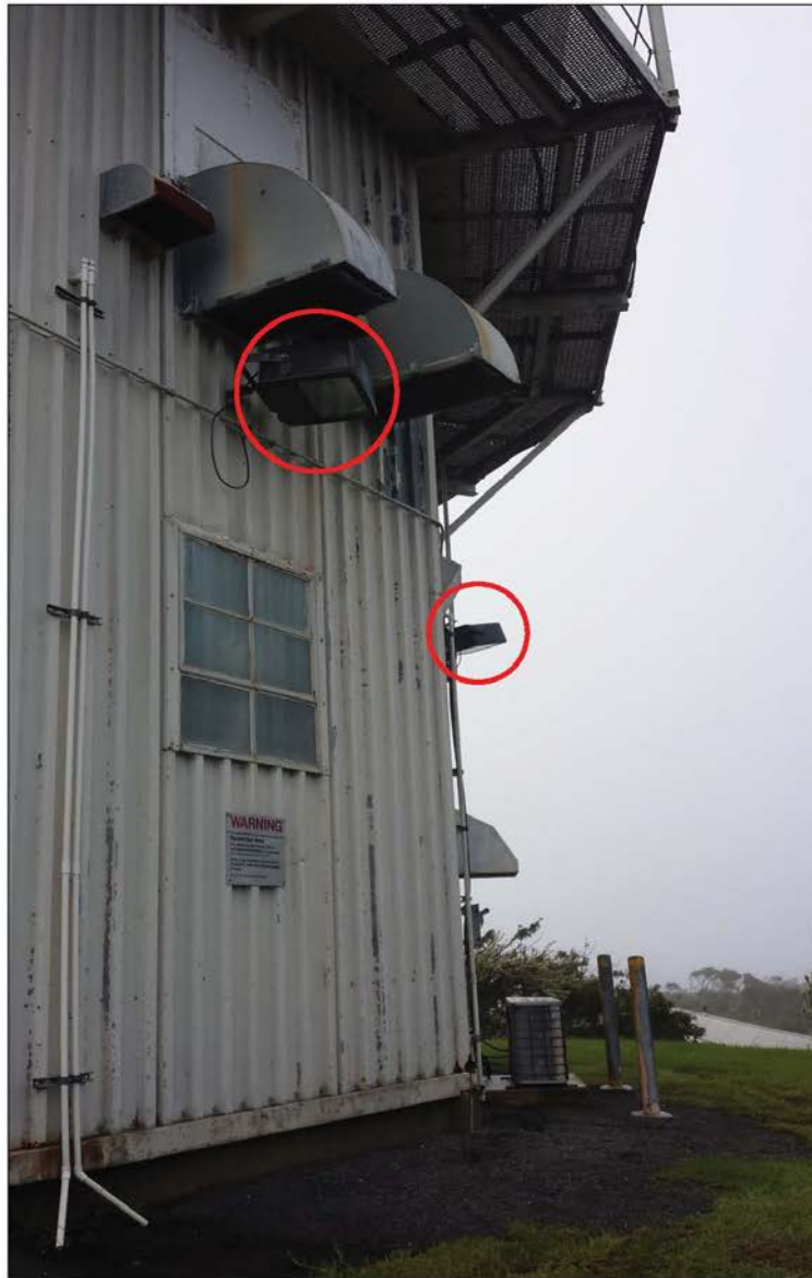
Perimeter Light_I: One green bulb, with full shielding (circle on the left)
