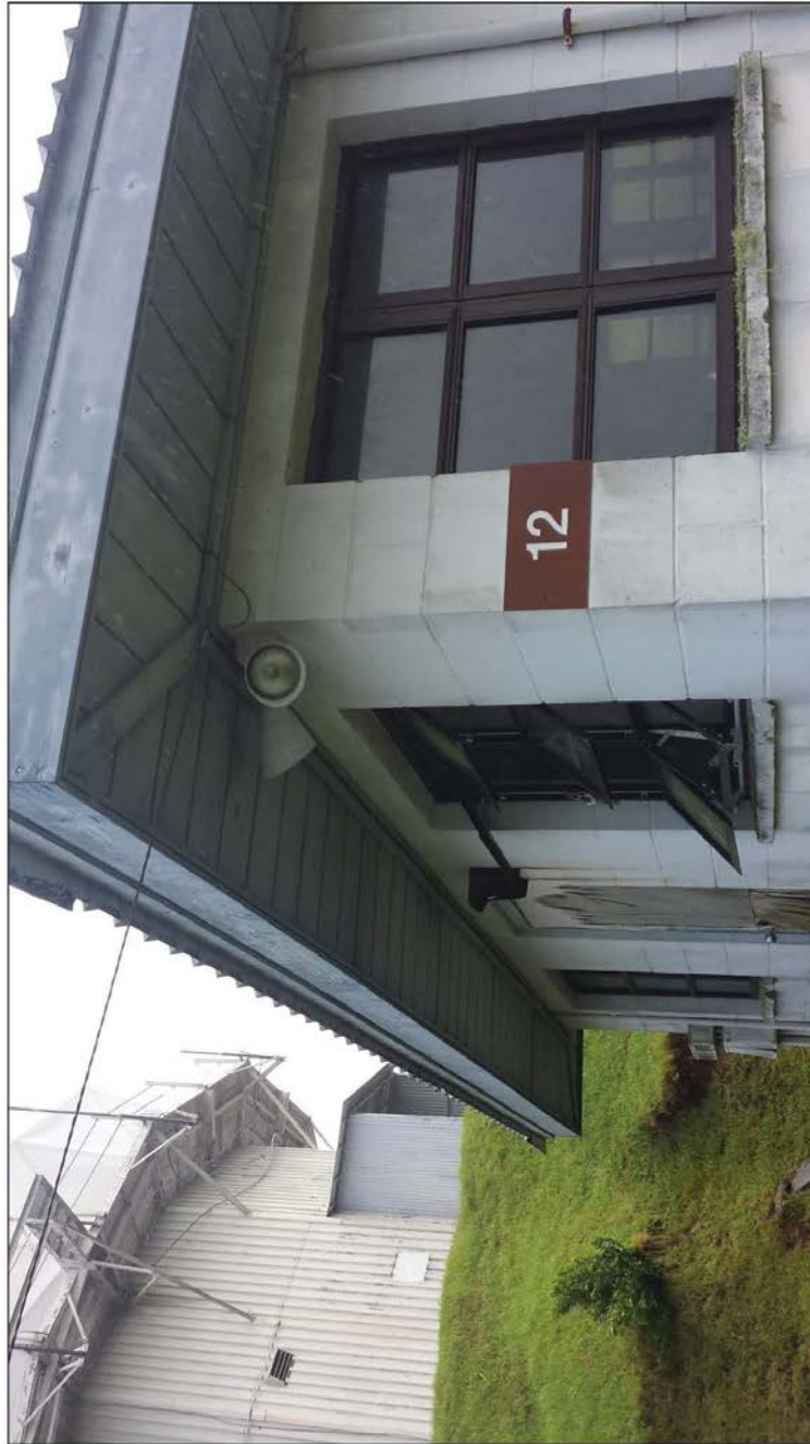
Building 12_Flood Light 1: Two white bulbs each with shielding and no motion detection (building appears to no longer be in use).
