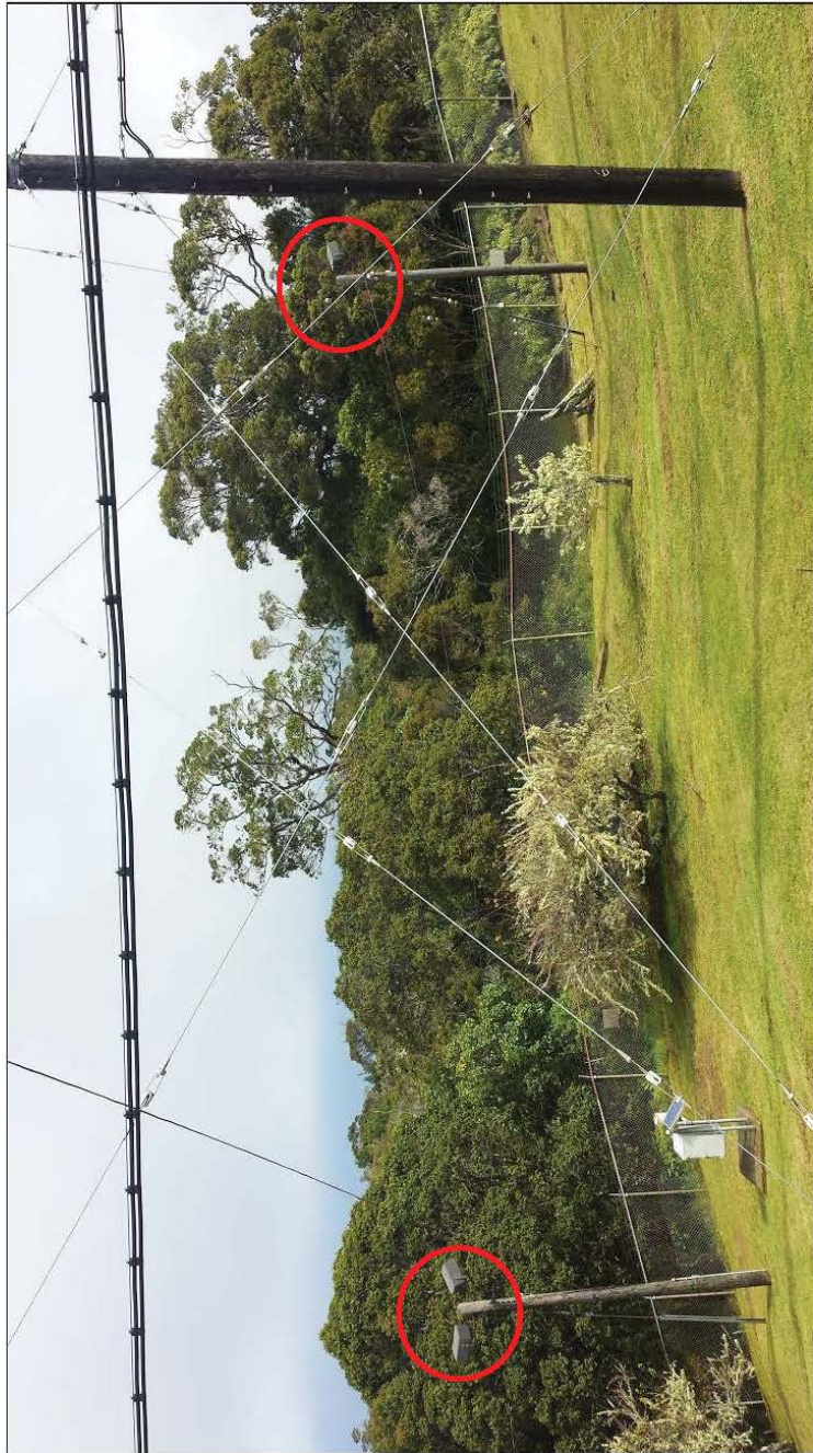
Perimeter Light_E : One green bulb, with full shielding (circle on the right)
