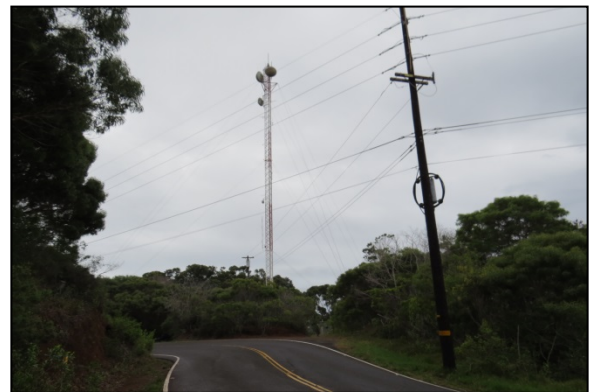
Looking south on Rt. 550 at Kōke`e MAS
