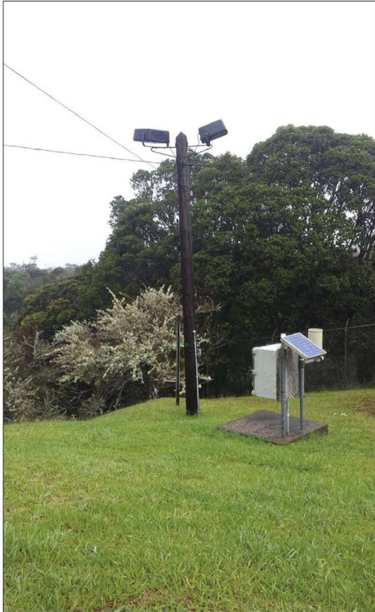
Perimeter Light_F: Two green bulbs, with full shielding.
