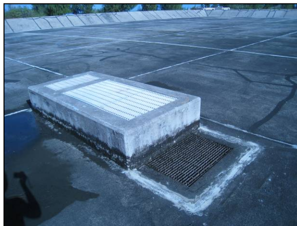
Inlet for Outfall No. 3
