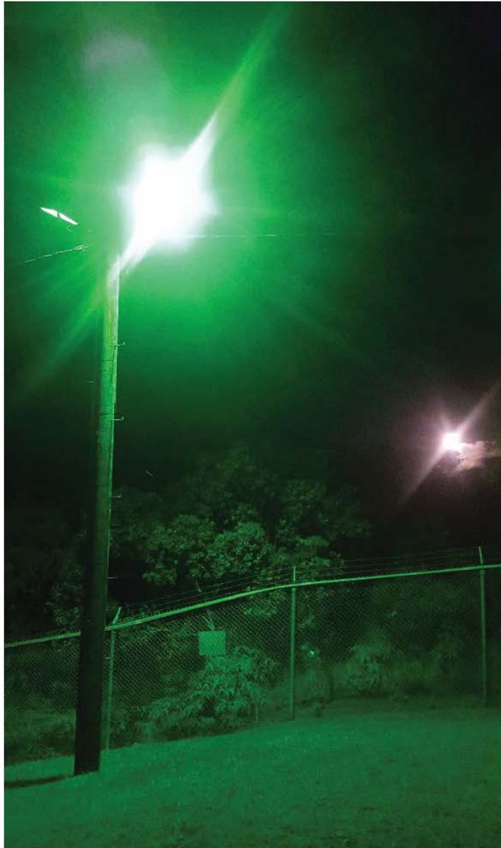
Perimeter Light_D: One green bulb, with full shielding (moon is visible in the background).
