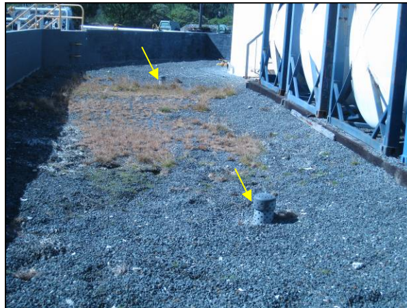
Inlets to Outfall No. 5
