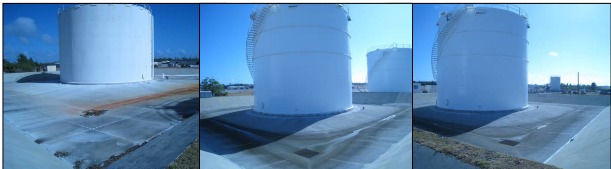
Inlets to Outfall No. 6
