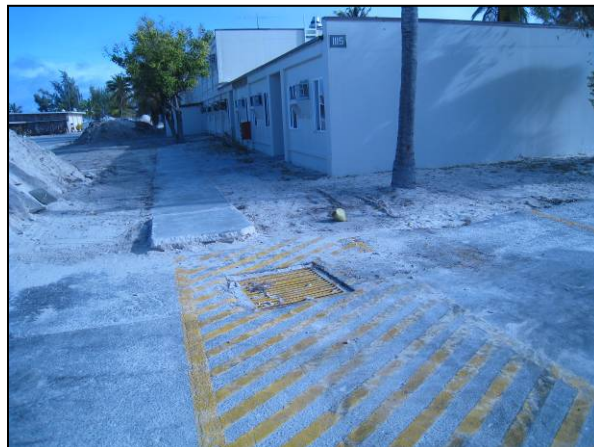
These photographs show the inlets on the southwest and southeast corners of Building 1116 (Medical Clinic).
