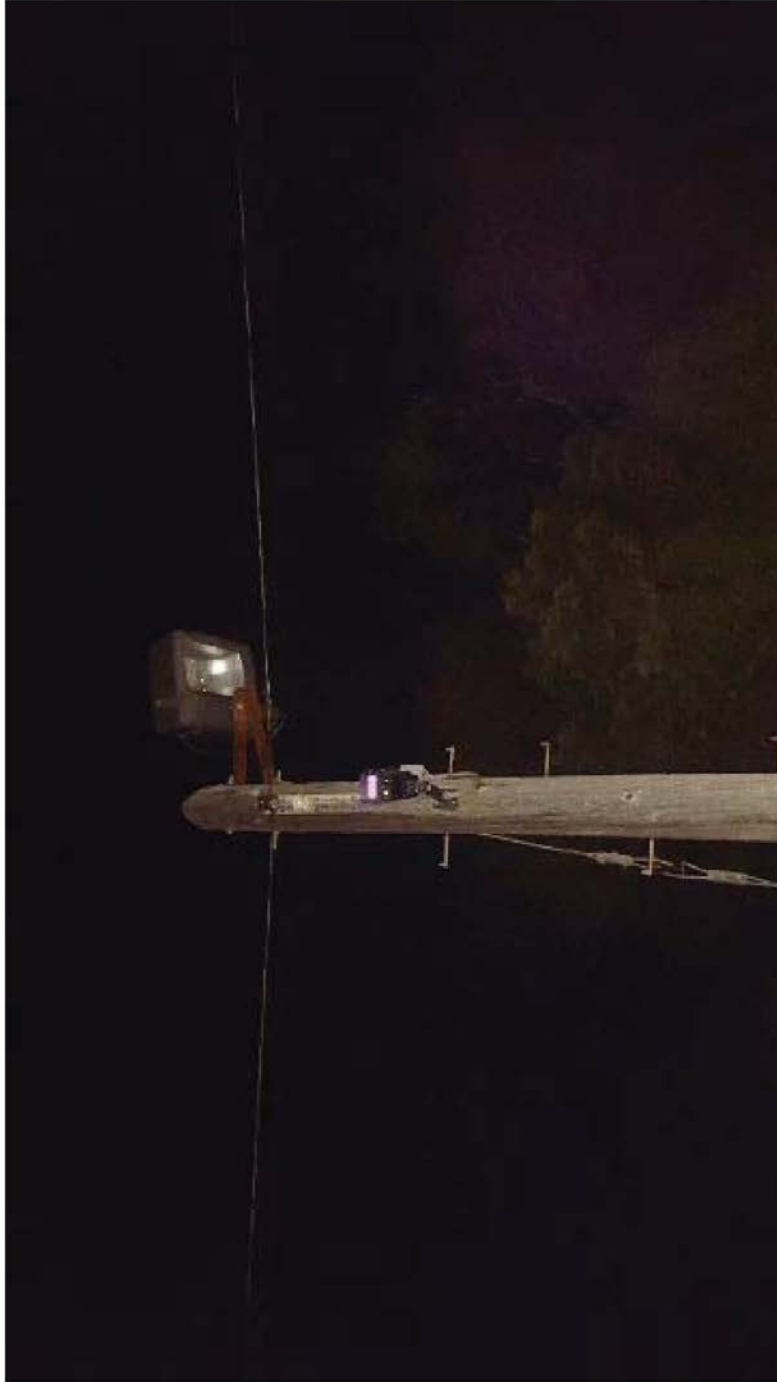
Perimeter Light_E (close up): One green bulb, with full shielding, light is currently not functioning.
