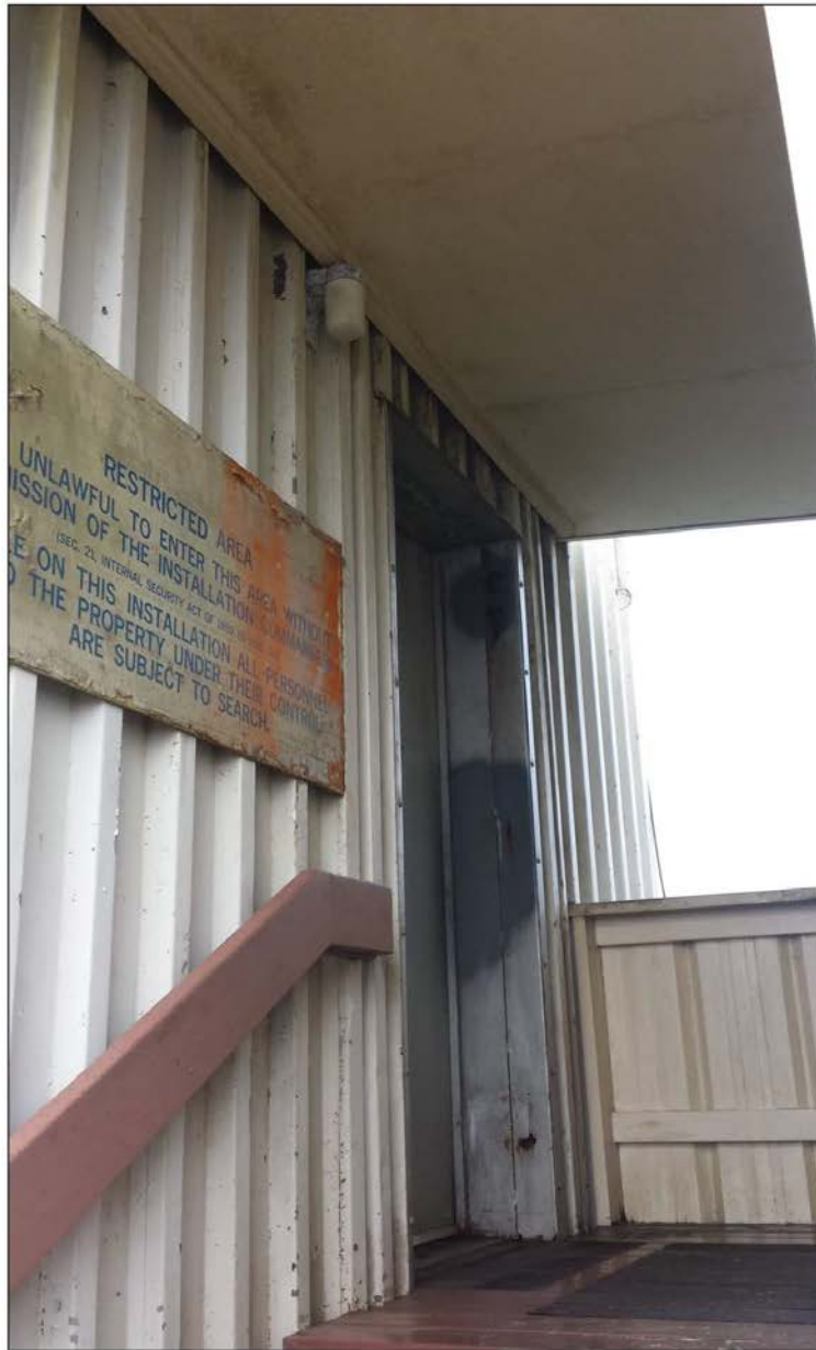
RadarTwr_Entryway Light 2: One white bulb with no shielding and no motion detection.
