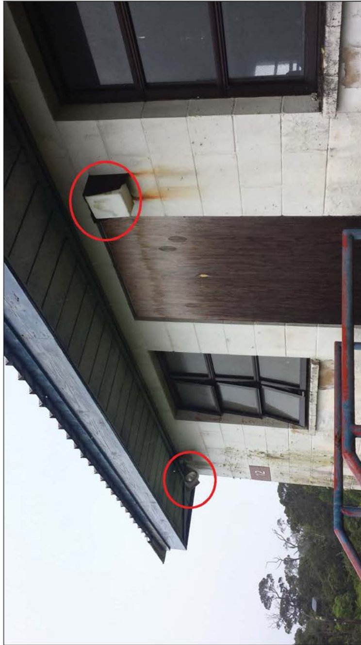
Building 12_Flood Light 2 and Entryway Light 1: Three white bulbs each with shielding and no motion detection (building appears to no longer be in use).
