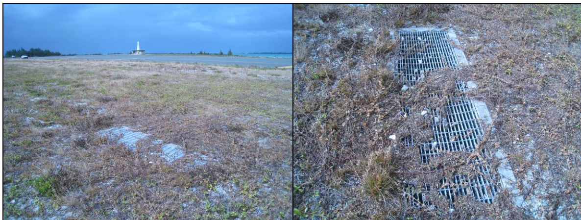
Inlet for Outfall No. 4
