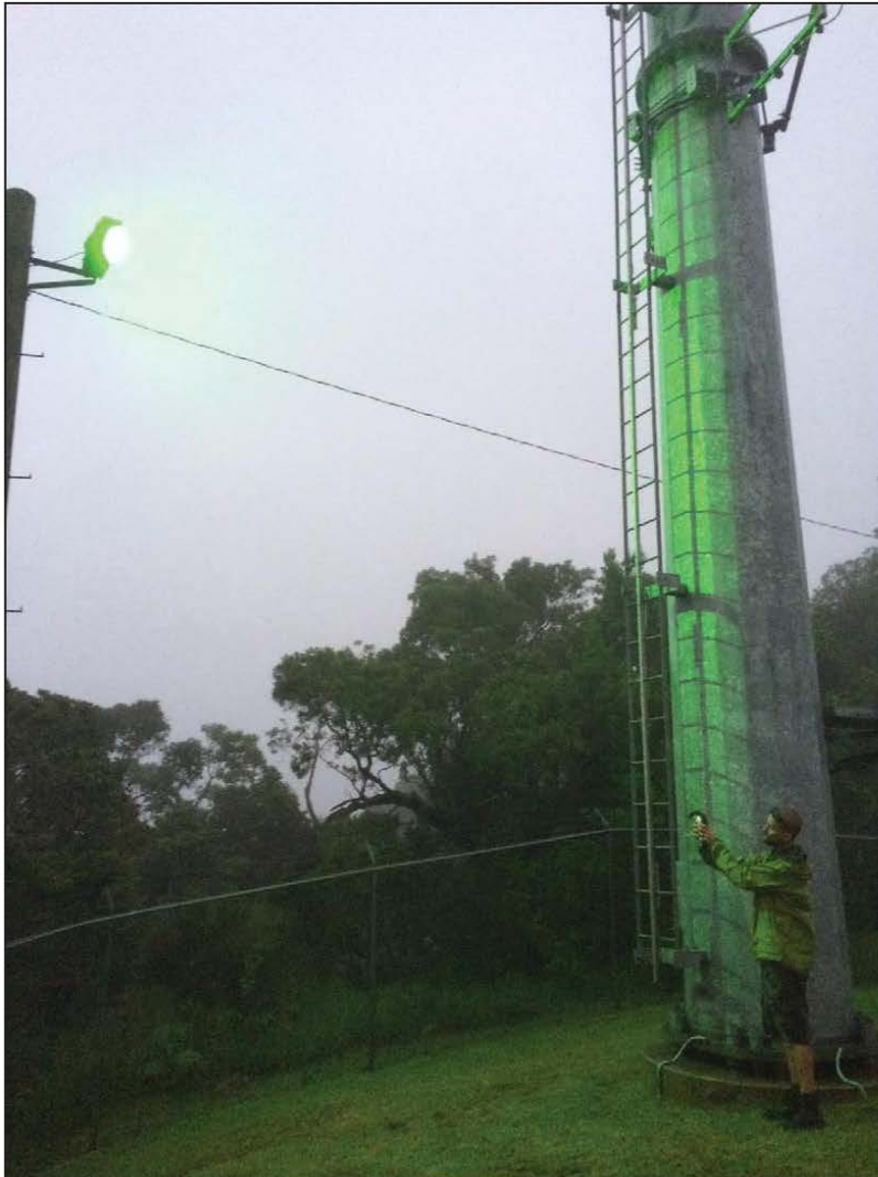
Perimeter Light_C: One green bulb, with full shielding (photo taken before the light was realigned in a downward position).
