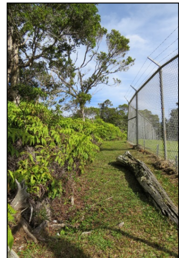
View along the fence line in Kōke`e HMU-2
