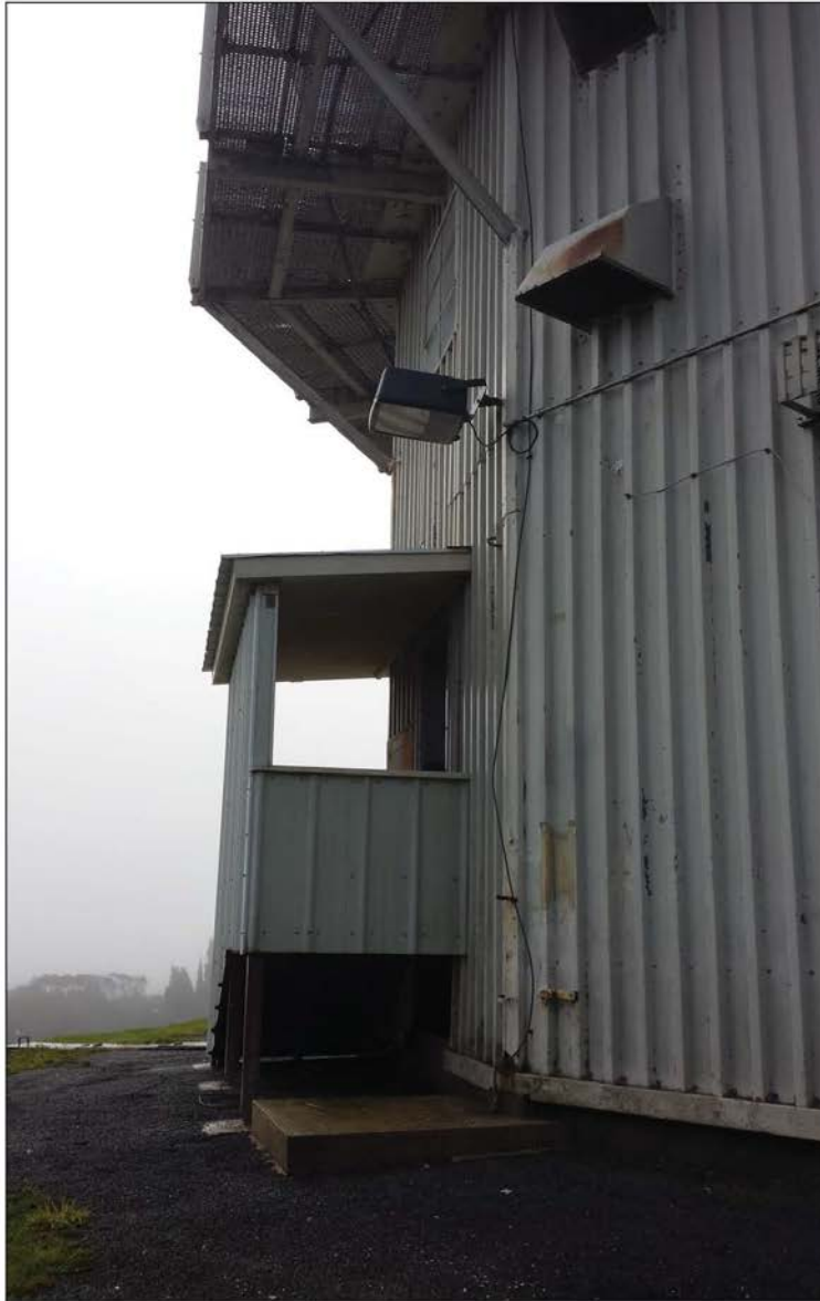
Perimeter Light_H: One green bulb, with full shielding, mounted to the Radar Tower building.
