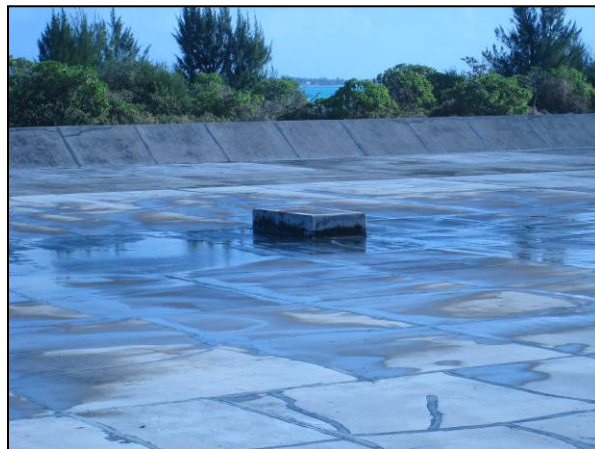
Inlet for Outfall No. 2
