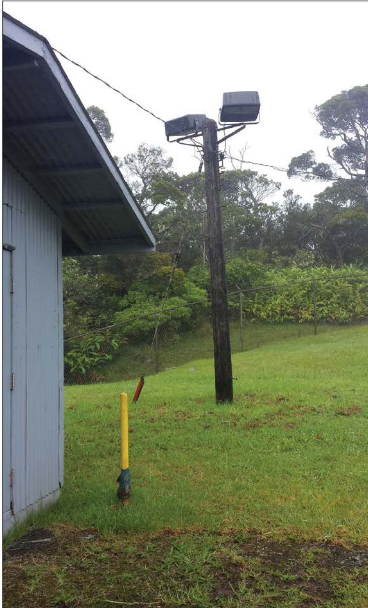
Perimeter Light _M: Two green bulbs, with full shielding, immediately west of building 6.
