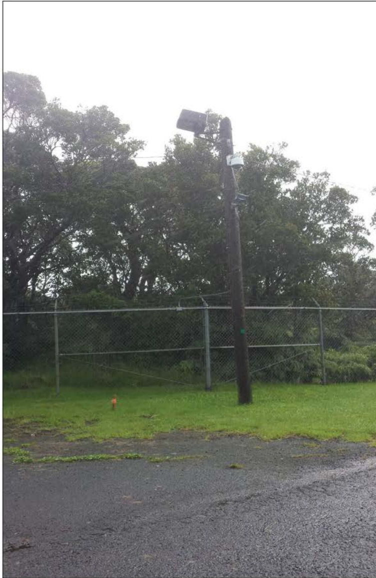
Perimeter Light_B: One green bulb, with full shielding (close up).
