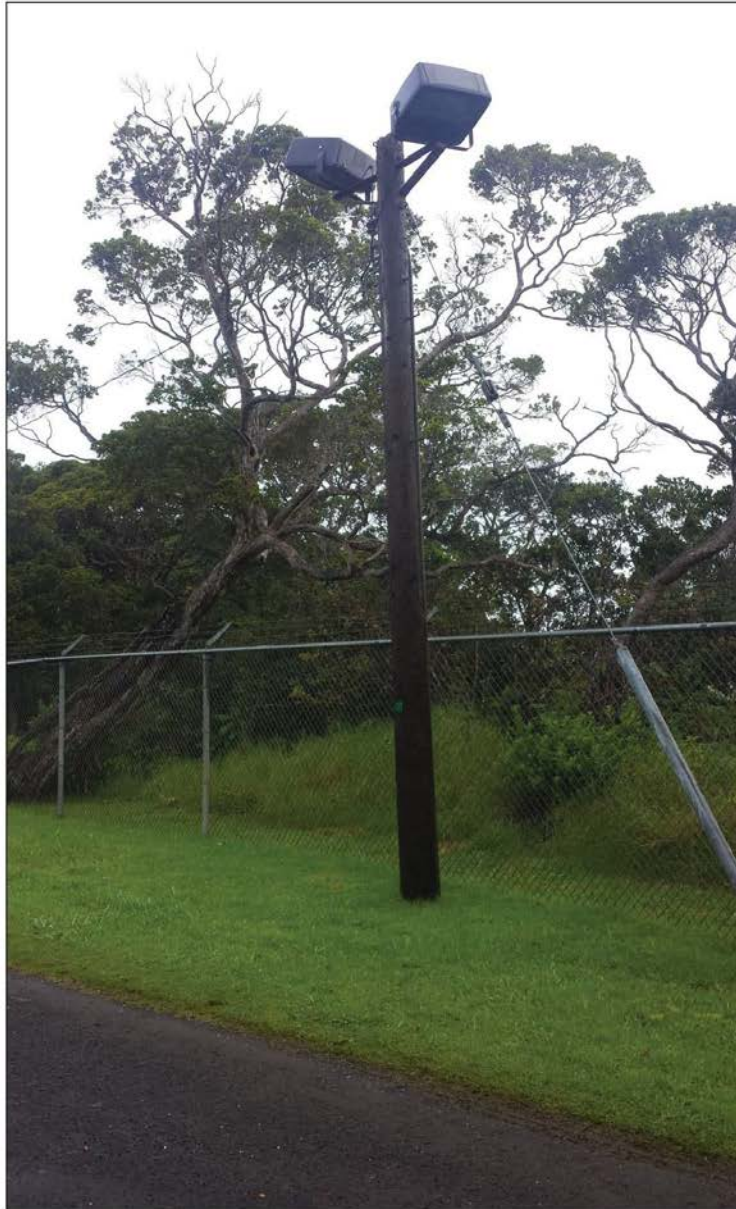
Perimeter Light_A: Two green bulbs, with full shielding (close up).
