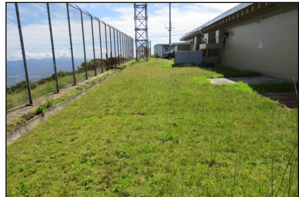
Mowed and maintained vegetation on Mt. Ka`ala AFS
