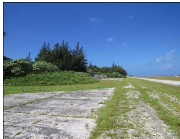
Looking west along the north side of HMU-15
