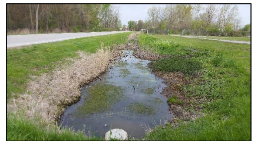
Storm water conveyance area
