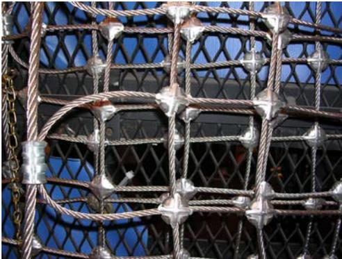
Figure 3: Star and Cylindrical Fasteners
