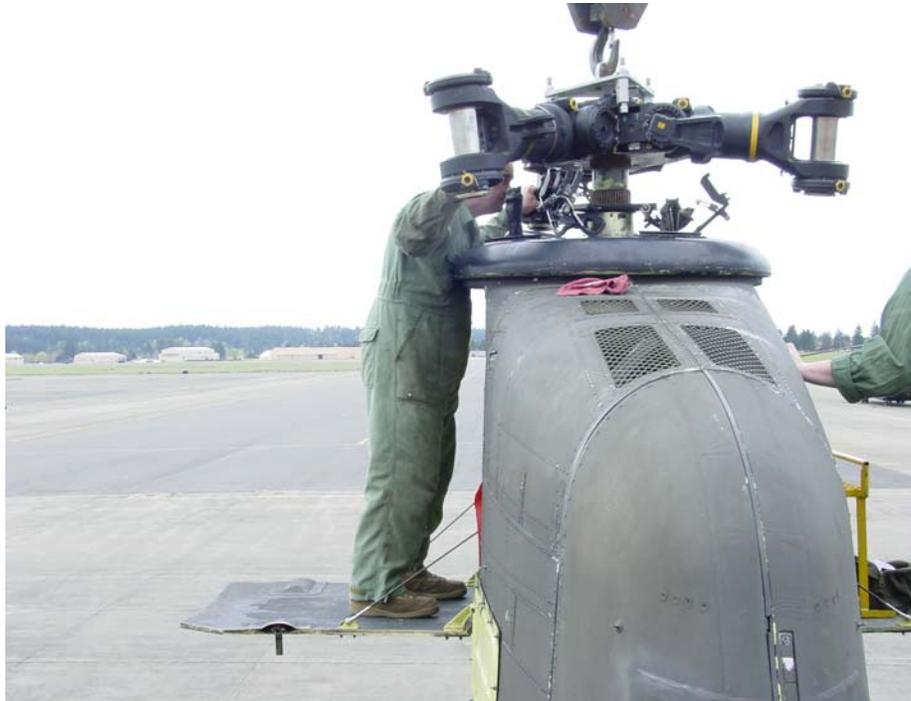
SSG Steven Stretch guiding in the aft rotor head. Notice his height in relation to the aft rotor head.
