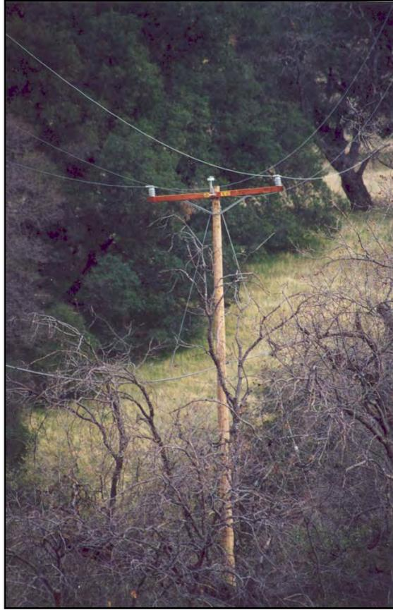
**Figure 15. Avian-safe Structure with 60-inch Conductor Separation**
