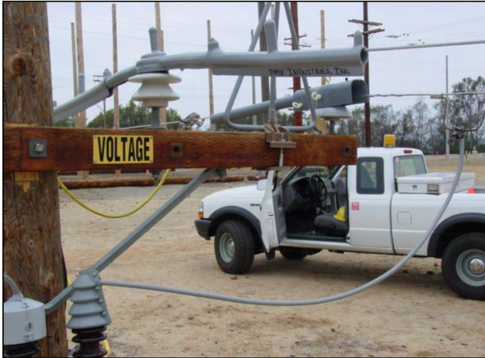
Figure 18. Pin and Insulator Covers, Transformer Bushing Covers and Jumper Coverups
