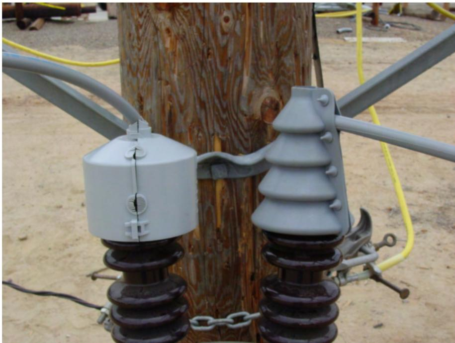
Figure 19. Transformer Bushing Covers and Jumper Coverups
