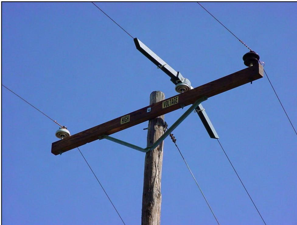
**Figure 22. Pin and Insulator Cover**
