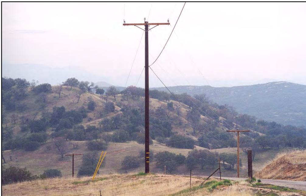
**Figure 14. Avian-safe Structure with 60-inch Conductor Separation**
