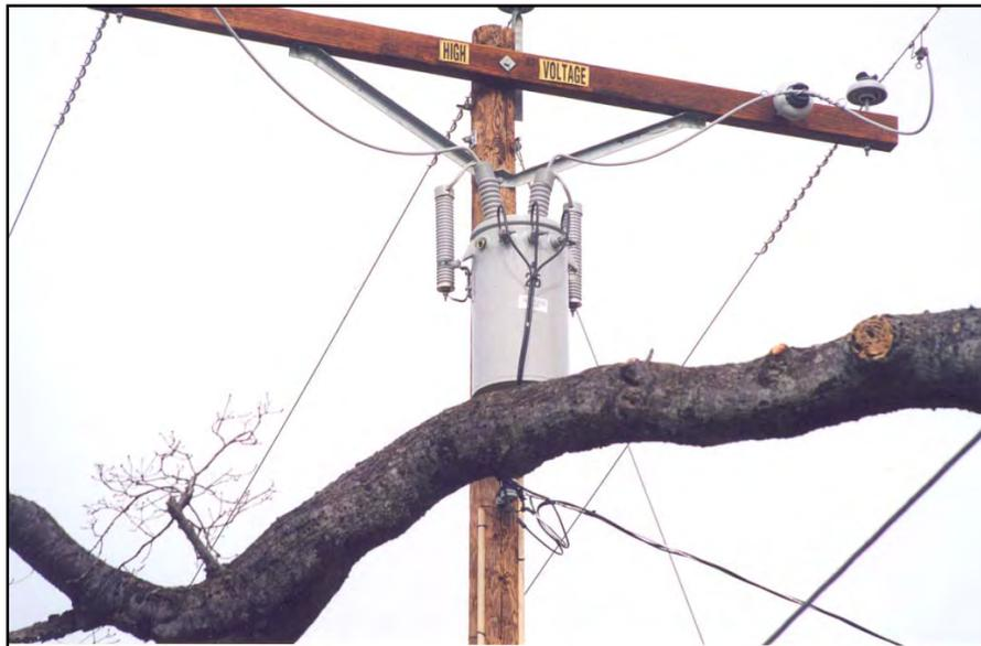
**Figure 17. Bushing Covers, Lightning Arrester Covers and Jumper Covers**
