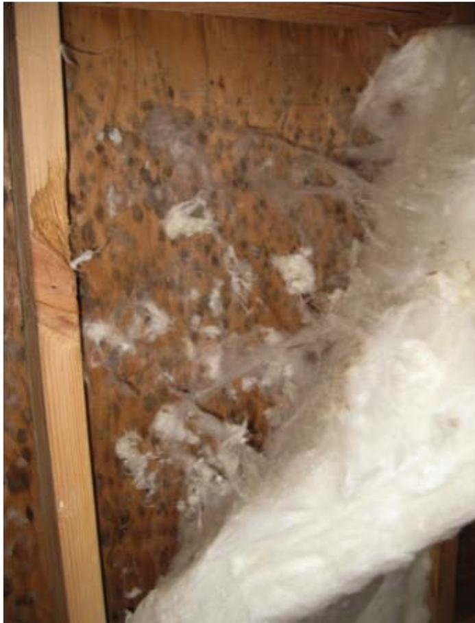
Sealing air leakage can create indoor air quality problems by allowing excess humidity and pollutants to build up. Air sealing must be coupled with ventilation to ensure healthy indoor air quality.
