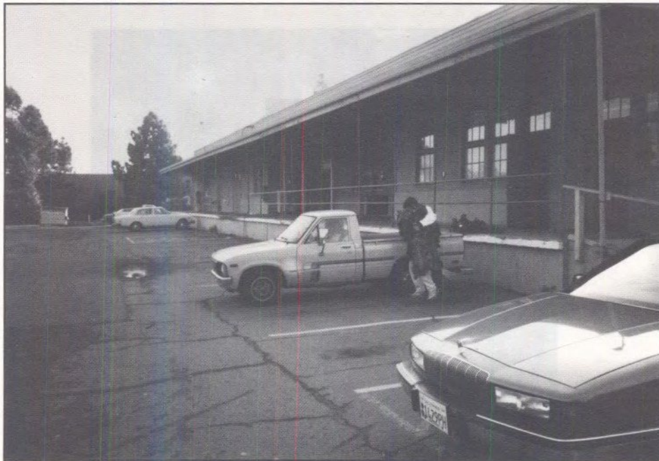
Figure 34. Exterior view of Repository #2.
