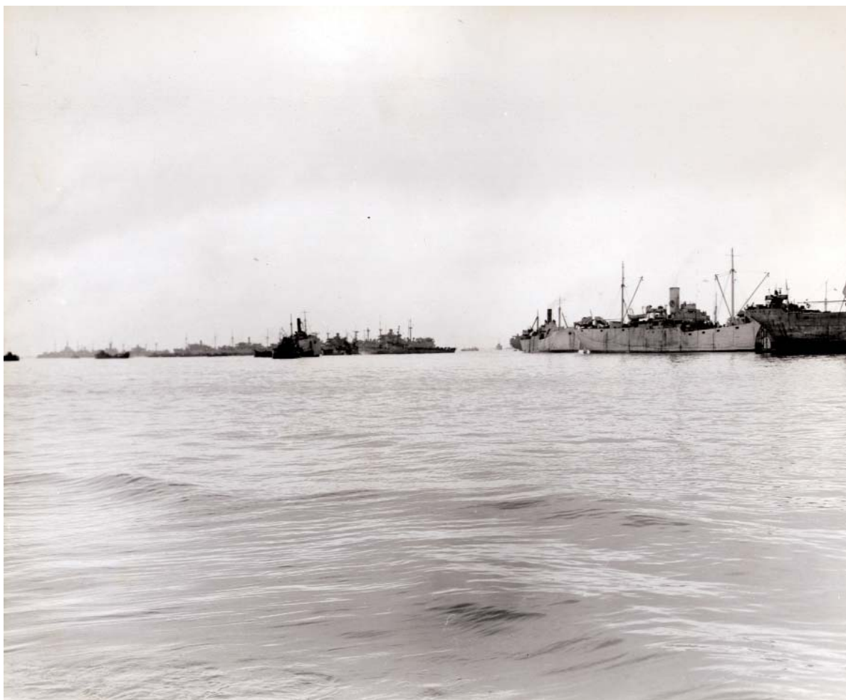
Above: The Gooseberry line of sunken ships (National Archives Photograph No. 80-G-284124).
