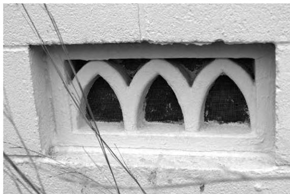
Figure 56. Crawl space vent openings must be small enough to prevent placement of hand-carried explosive devices beneath buildings (ERDC-CERL 2002).
