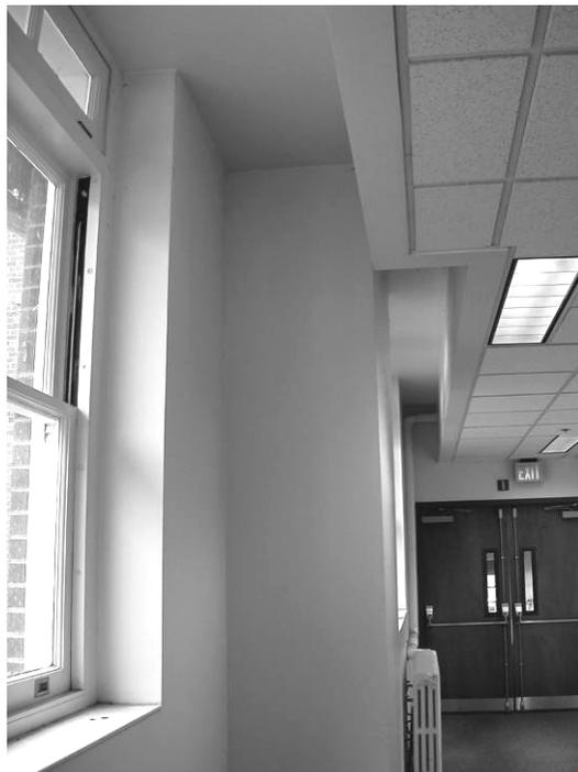
Figure 47. Ceilings dropped to accommodate new ductwork should be pulled away from historic fenestration. Historic radiators and operable windows and transoms should be retained (ERDC-CERL 2004).
