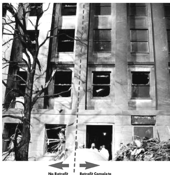
Figure 39. Pentagon immediately after September 11, 2001, showing intact blast-resistant windows at right (DON 2001).
