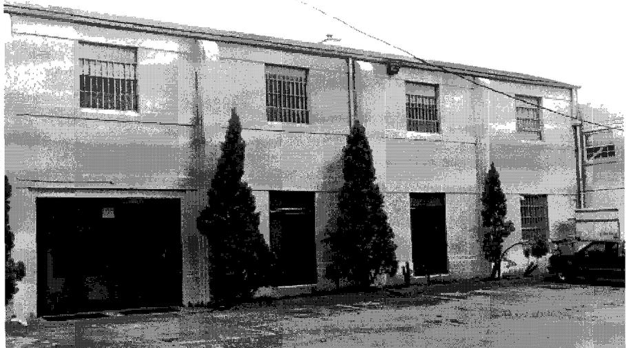
With art classes planned inside, the architect for the remodeling project called for large windows to be added to the building's north side. Installation of the modern windows required the contractor to slice through several inches of reinforced concrete.
