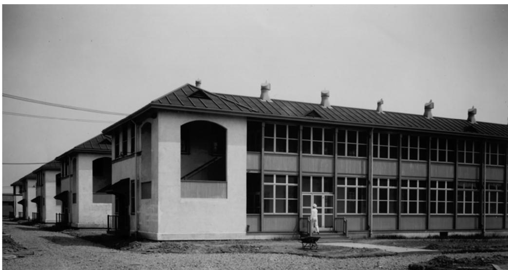
Figure 235. Enclosed porches and open staircases on the wards at the Philadelphia Navy Yard Emergency Hospital, Pennsylvania, June 1919 (NARA College Park, RG 71-CA, box 389, 2854).
