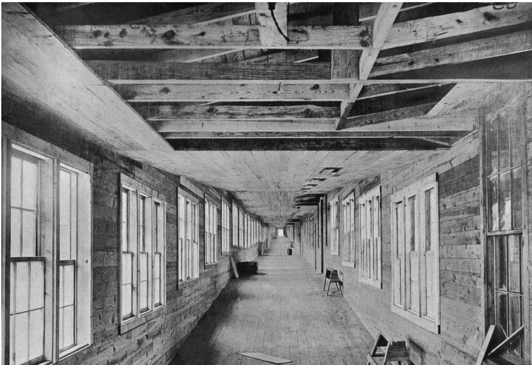
Figure 216. Interior of connecting corridors at a WWI hospital under construction, circa 1918, Camp Upton, Yaphank, Long Island, New York (National Army Cantonments).
