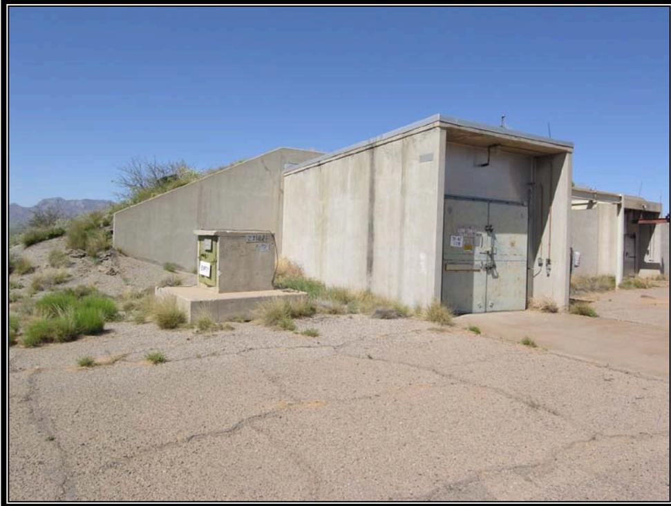
Plate 8.9 The large structure is a climatic test chamber for various munitions. The small structure to the left is a nine square foot magazine (Courtesy U.S. Army, 2007)
