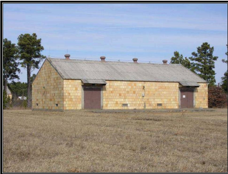
Plate 6.8 Typical powder magazine (Courtesy U.S. Army, 2007)
