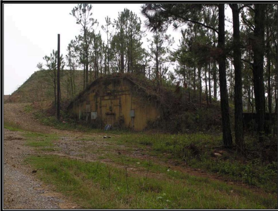
Plate 7.25 Typical installation-level magazine for fuze and detonator storage (Courtesy U.S. Army, 2007)
