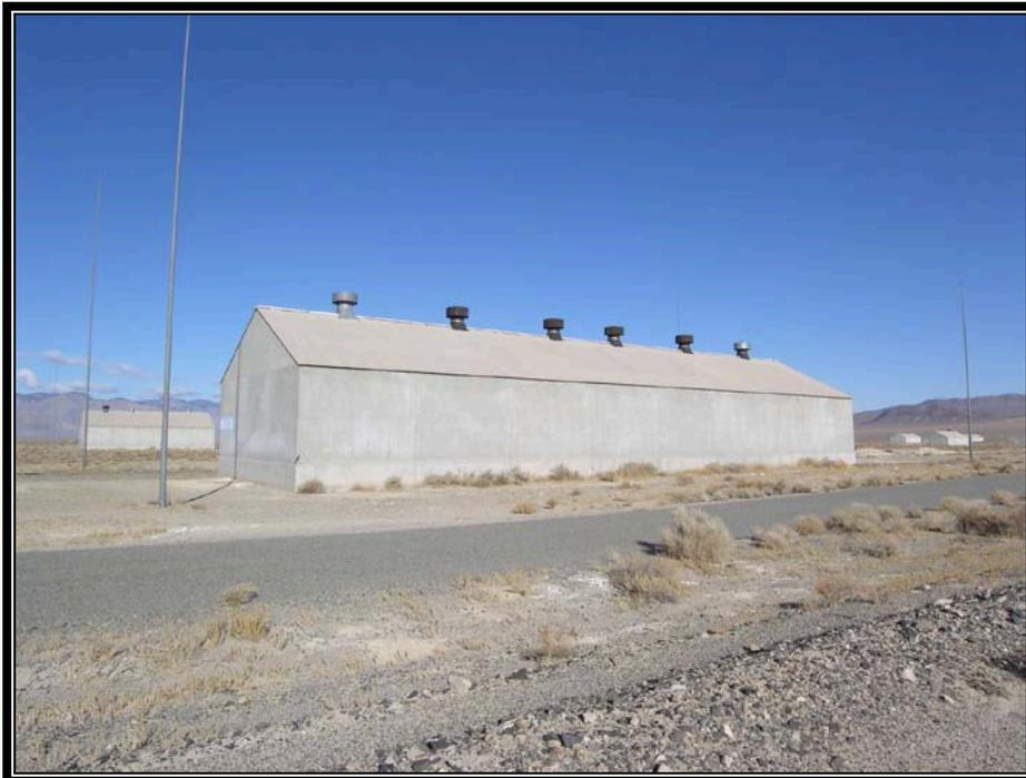
Plate 6.29 Typical group lightning protection for aboveground magazines (Courtesy U.S. Army, 2007)
