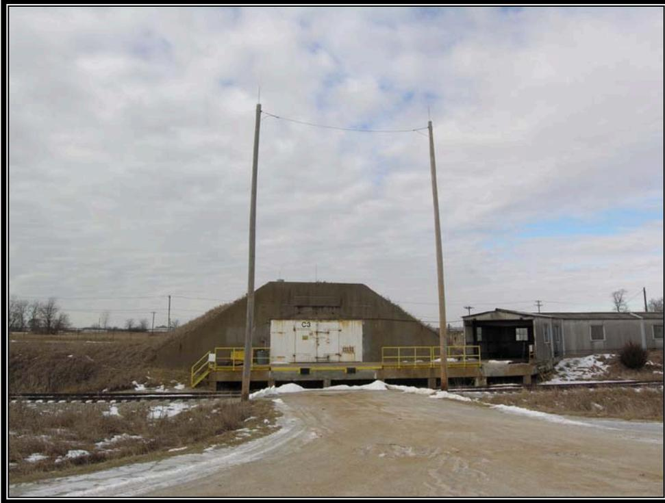
Plate 6.30 Typical shielding system of lightning protection at igloo storage (Courtesy U.S. Army, 2007)
