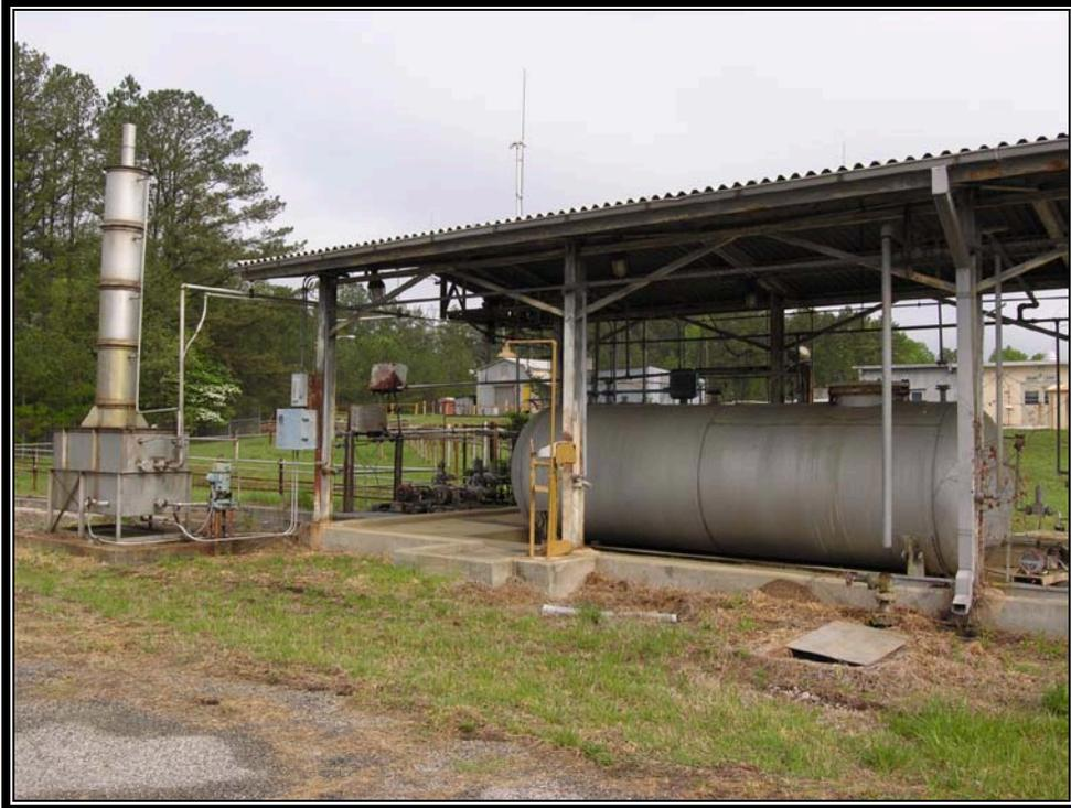
Plate 7.8 Typical storage tank and shelter for inhibited red fuming nitric acid (Courtesy U.S. Army, 2007)
