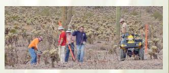
RMO personnel installing bright orange plastic poles in the primary impact zone. The poles provide a buffer without compromising site location information and are highly visible to EOD personnel for avoidance when traversing the range, providing protection from inadvertent vehicle damage.
