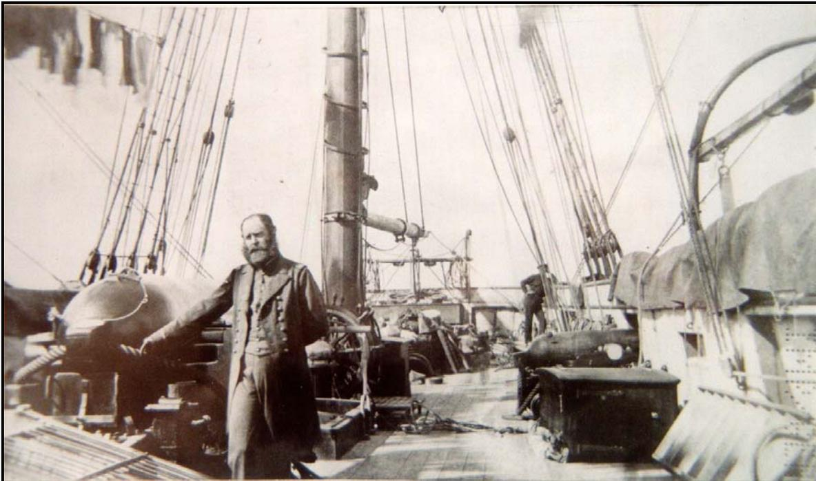
**Figure 28. Kell at the aft pivot gun and a Fawcett, Preston and Company 32-pounder on the port quarter.**
