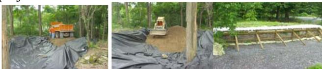
Further treatment depends on the feature's need for further stabilization. In severe situations stabilizing structures may be added. This residence in Sterlingville is an example. Sometimes honeycomb material is used to keep the sand and/or gravel in place. Other properties were
