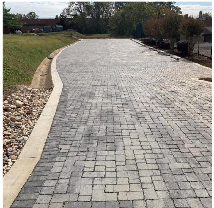
Permeable pavers replaced deteriorating asphalt in an overflow parking area on base.
