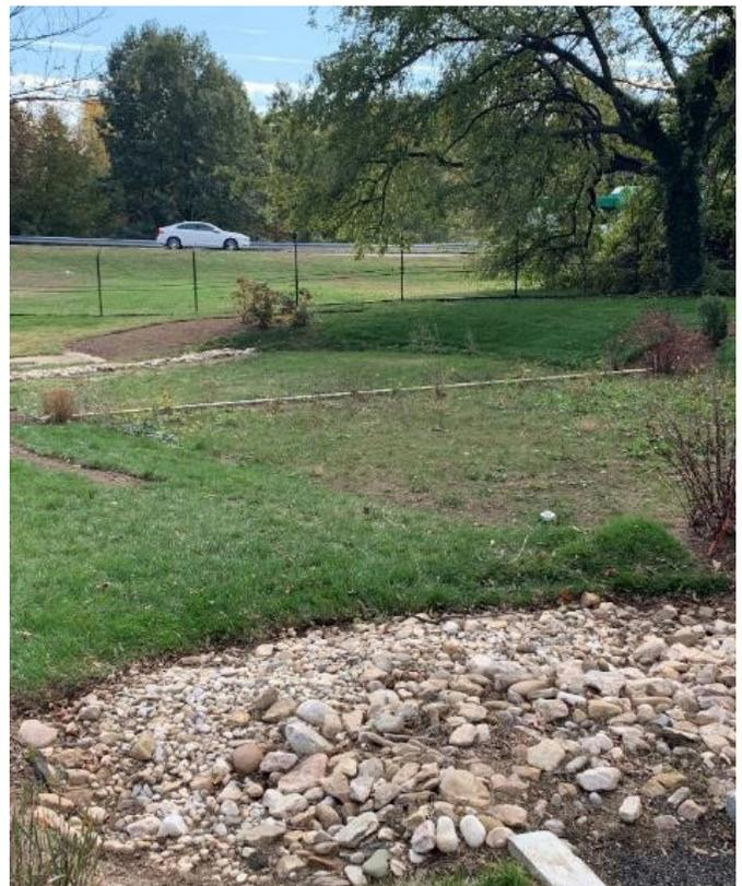
*The two-tiered bioswale uphill from an outfall, collects stormwater from paved parking lots and roadways.*
