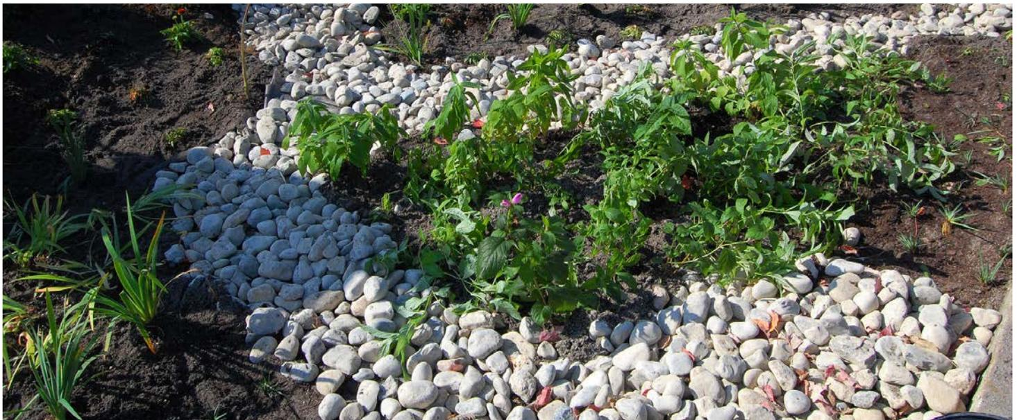
Changes to the design of bioretention cells, such as the one shown here, can enhance the infiltration or nutrient removal that occurs in the system.
