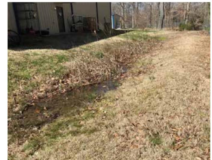
Operational issues, like the clogged media caused by prolonged ponding shown here, can be prevented or resolved through routine maintenance and inspection.
