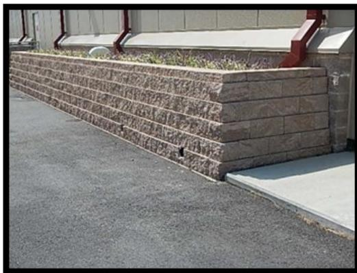
Disconnected roof drains at Naval Station Norfolk.
