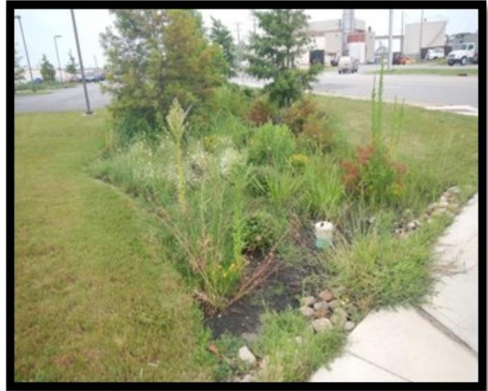
A bioretention area BMP at Naval Station Norfolk.
