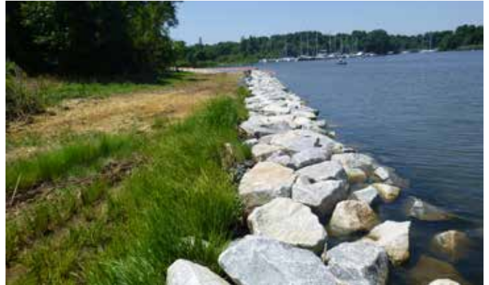
Possum Point shoreline after restoration
