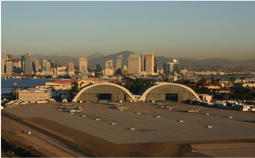
Naval airstation hangars in San Diego . (Getty Images)
