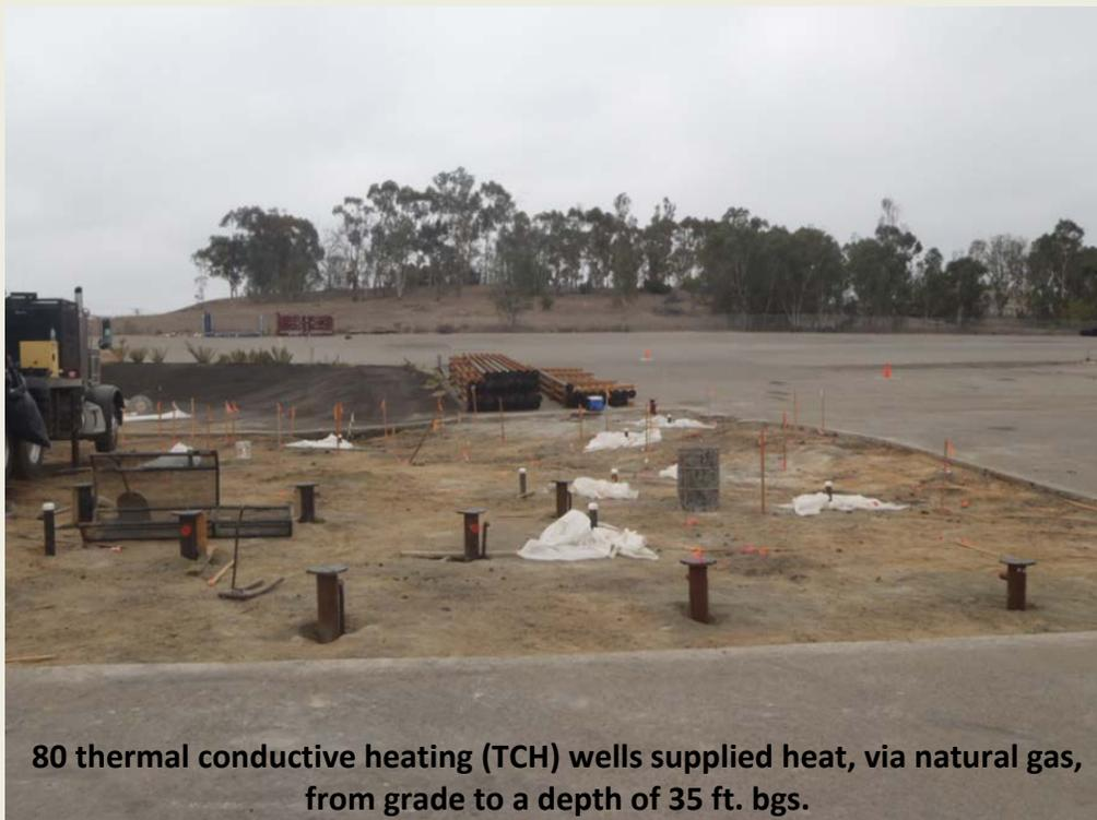
**80 thermal conductive heating (TCH) wells supplied heat, via natural gas, from grade to a depth of 35 ft. bgs.**
