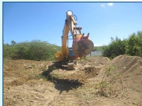
*Figure 8: Magnetic attachment on excavator removing bombs from the roadbed. In areas where it is too dangerous and/or too costly to remove munitions by traditional methods, remotely operated equipment has been shown on Vieques to significantly reduce explosive hazards to workers and cut costs by more than half.*
