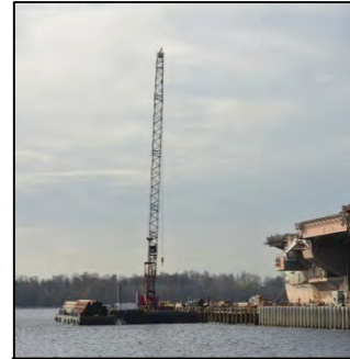
Figure 10: Pier 4 being repaired.
