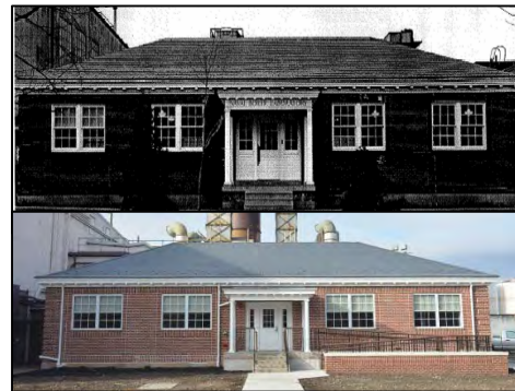
Figure 11 Building 531 in 1939 (top) and (2015) following rehabilitation (bottom). Note the addition of the wheelchair ramp on the right side.
