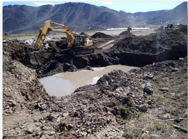
**Photo 3:** Soil excavation activities at the Main Operations Complex, showing groundwater accumulating in the excavation. View south towards Kangukhsam Mountain. (7/2013, J. Craner)
