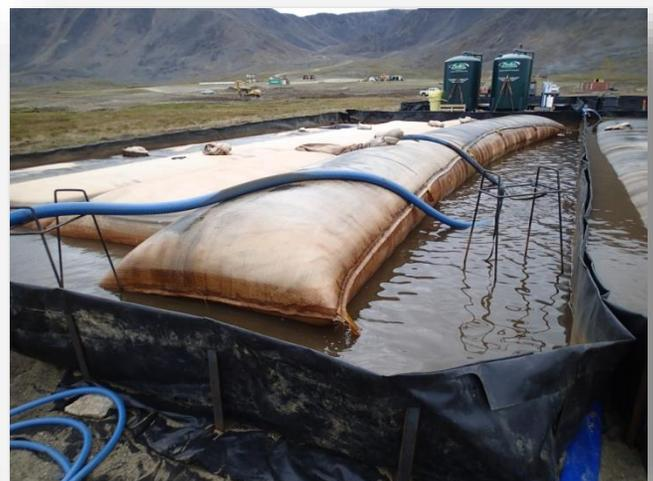
**Photo 6:** Geotubes being filled with sediment/water/flocculant slurry, slowly dewatering into containment areas. Two large GAC units used as final water treatment step prior to discharging to ground surface. Main Operations Complex in background facing south. (9/2013, J. Craner)
