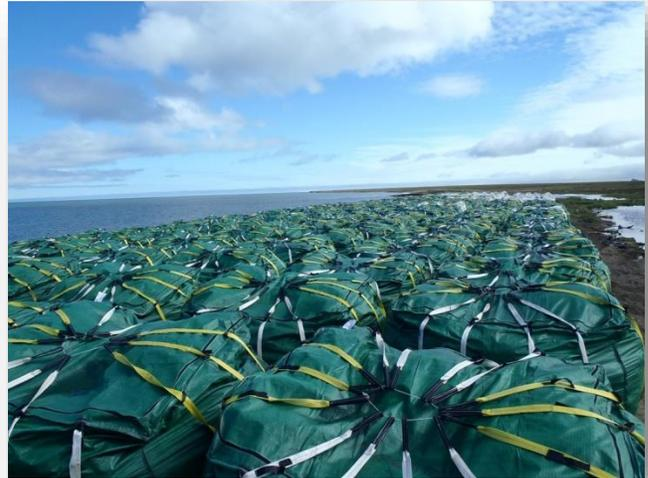
**Photo 2:** Over 600 bulk bags are staged at Cargo Beach for transportation offsite via barge. 9 cubic yard bulk bags used to containerize petroleum and PCB-contaminated soil for disposal in the lower 48. View east along the beach. (9/2013, R. Broyles)
