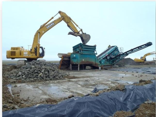
**Photo 4:** Screen plant operations at soil stockpile management pad. Oversized gravel separated into piles for use as backfill, avoiding offsite transportation and disposal costs. (7/2014, J. Craner)
