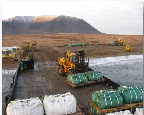
**Photo 1:** Loading the Sam Talaak landing craft barge with 9 cubic yard bulk bags of contaminated soil staged at Cargo Beach. View south towards Kanguksam Mountain and the Northeast Cape site. (8/2013, R. James)
