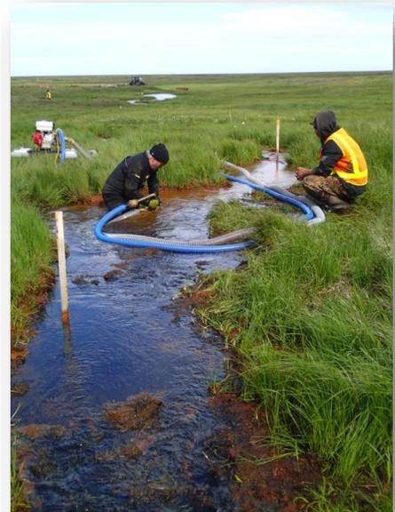
**Photo 5:** Bristol employees Johnny Willis (left) and Albert Kulowiya (right), operate the sediment suction dredge (top left) to remove loose sediment from the wetland. Sediment/water slurry was pumped upslope, flocculant added, transferred to geotextile tubes for dewatering, and excess water treated with GAC units before discharge to ground surface. (8/2013, J. Craner)
