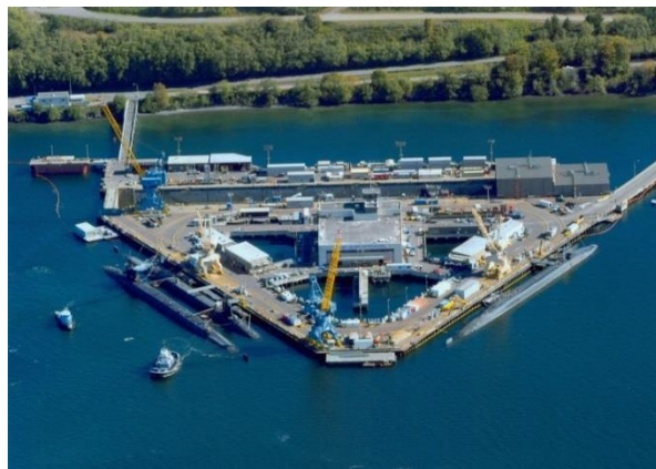
Photo of the Delta Pier at NAVBASE Kitsap Bangor
