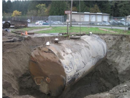
Removal of 30-year-old single-wall steel Underground Storage Tank
