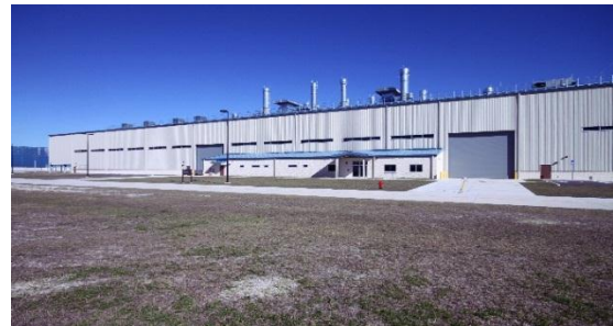
New Paint and Blast Facility at MCSF-BI
