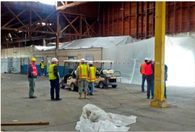
Warehouse asbestos abatement in progress.
