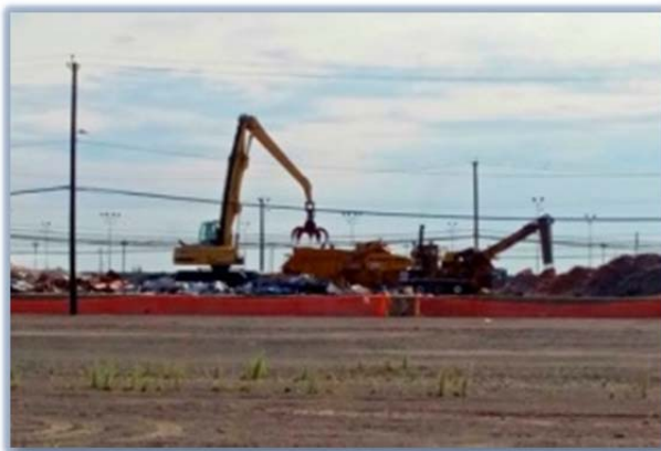
Warehouse demolition debris being loaded for shipment.
