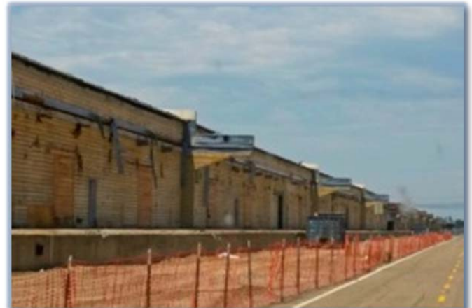
World War II-era warehouses with asbestos-containing siding removed prior to demolition.
