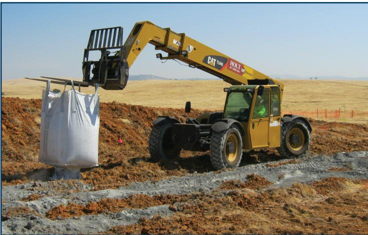
A stabilizer is added to lead contaminated soil at one of seven closed small arms ranges prior to tilling, excavation and truck loading. This prevents lead from leaching from the soil and allowed 638 truckloads to be disposed of at a Class II landfill less the five miles from the base and only 59 truckloads to be disposed of at a Class I landfill 200 miles away. After removal, local backfill soil was trucked in to restore the original land contours.
