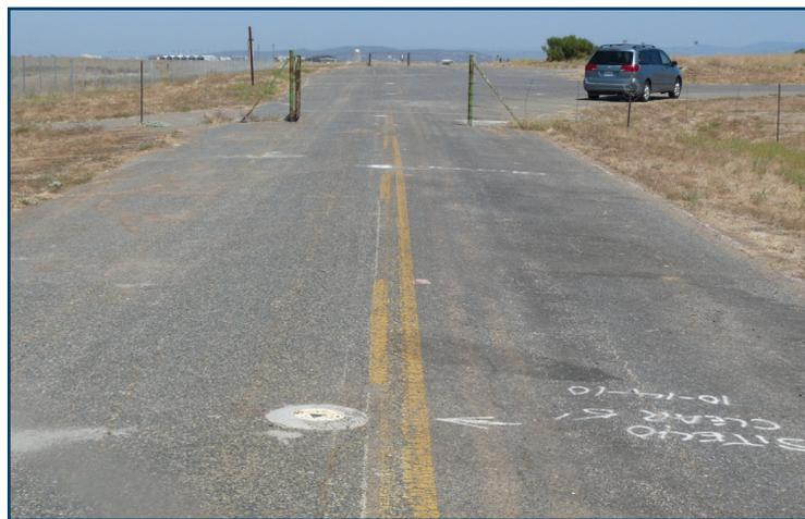
Hidden under five flush mount well caps are Emulsified Vegetable Oil injection points forming a biobarrier in a TCE contaminated plume at approximately 150 feet below ground surface. By 2013 the biobarrier has proven to be effective in cutting off the groundwater plume and preventing further migration into the runway security zone. A picket line of biobarrier injection wells can cut a contaminated groundwater plume in half shortening its life.
