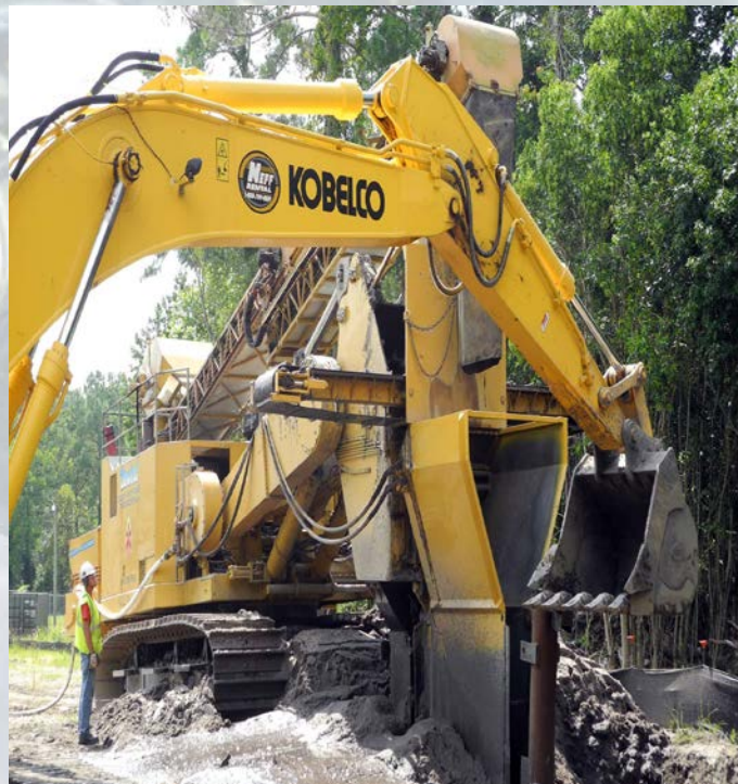
To address dissolved chlorinated solvents in groundwater underlying a major portion of the industrial area, a 600-foot long, 35-foot deep permeable reactive barrier was constructed using more than 700 tons of zero valent iron.
