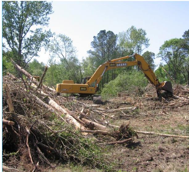
Heavily wooded sections of landfills were cleared, ground into wood chips and traded for compost. The cleared and graded landfill looks more like a park than a landfill.
