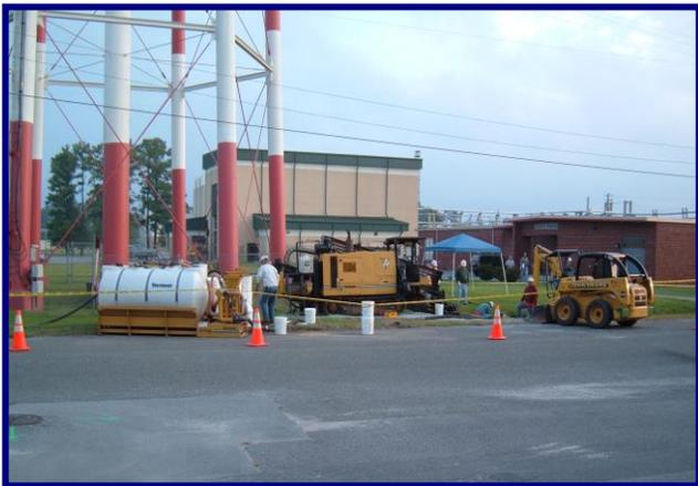
*Site 86 horizontal well installation. This successful technology has been implemented at two other locations at the Base. The sparging through a horizontal well was extremely effective with 99% contaminant reduction.*
