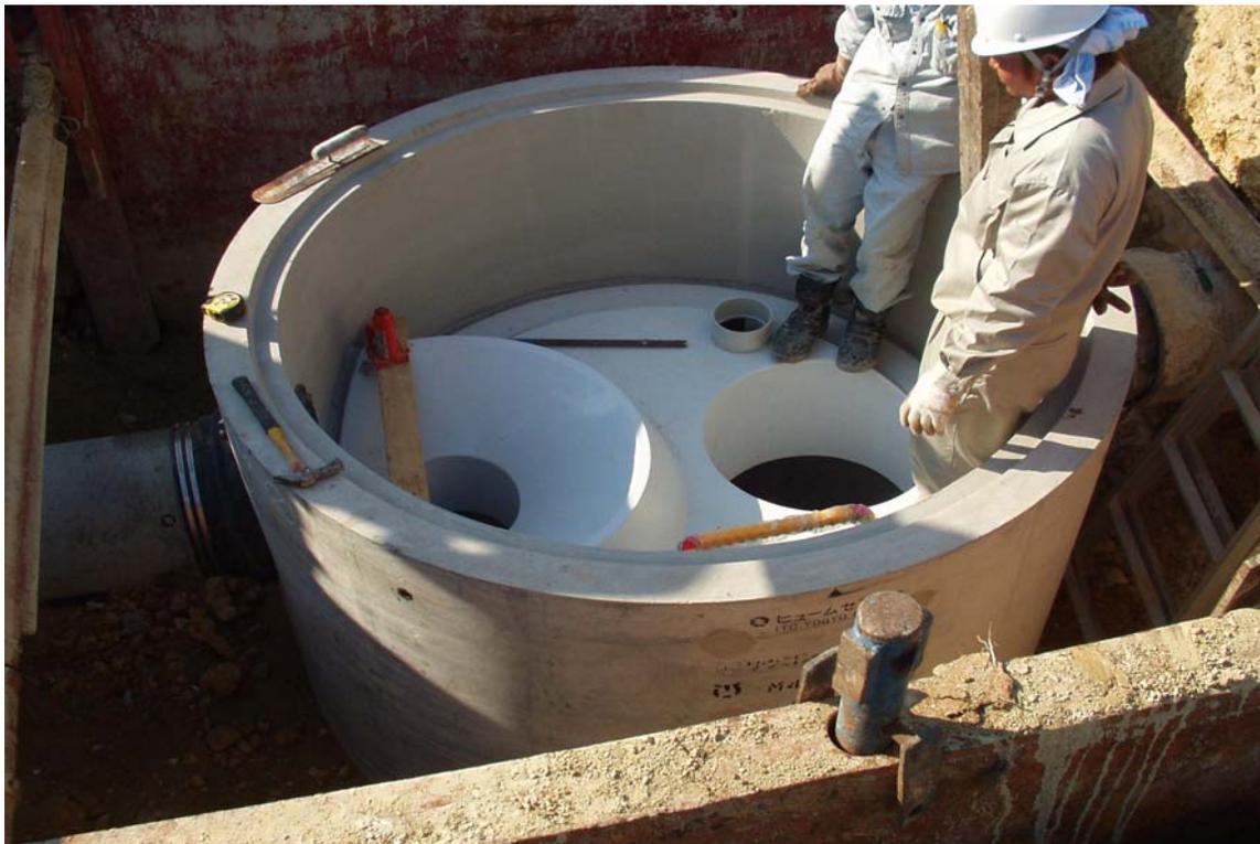
MCB Butler determined a need to alleviate stormwater discharges on Camp Foster. In 2005, ten sediment/oil separators using the high flow diversion weirs were installed. The diversion weir consists of a fiberglass insert that allows low flows containing stormwater pollutants to accumulate without being re-suspended during high flows.
