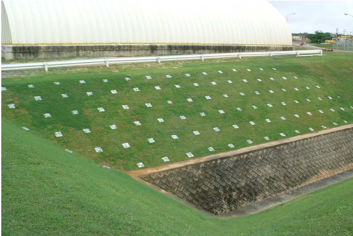
MCB Butler has selected soil nailing as the preferred method to deal with slope failures. As shown above, the repair of the slope at Camp Hansen was timely and cost effective. Soil nailing stabilized this foundation to ensure that the building was spared any permanent damage as the slope was secured.
