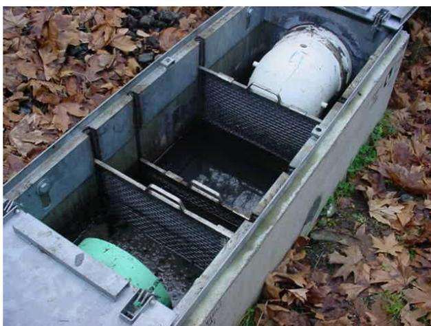
We also replaced old open top coalescing plate separators, which depended on the ability of floating weirs to remove oil, with new tank type separators which contain the residual oil and allow easy removal of the separated product.
