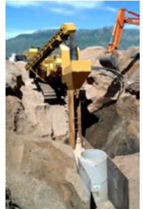
Contractors install a sump at OU1 as part of the groundwater collection system installed at the site.
