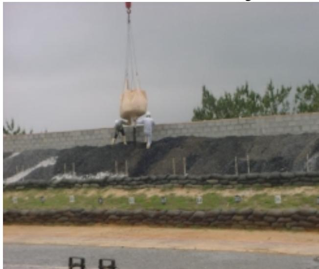
**Figure 7, Construction of Rubber Media Bullet Trap**
