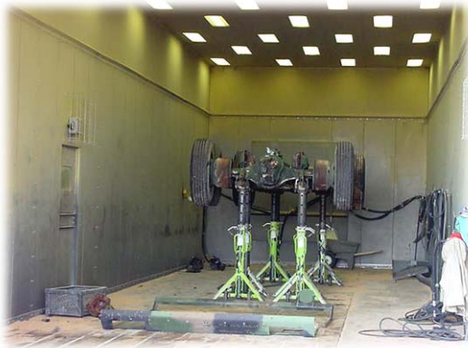
New paint booths helped to enable TXARNG to meet all minimum emission standards.
