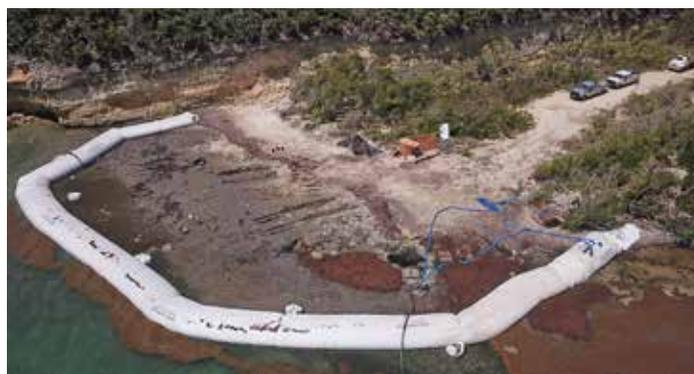
*Innovative use of a temporary, water-filled cofferdam significantly enhanced the safety and efficiency of operations to remove munitions located just offshore. The cofferdam allowed the site to be dewatered, such that UXO technicians successfully removed munitions without the need for UXO divers, thus accelerating the cleanup while increasing the safety of the operation.*
